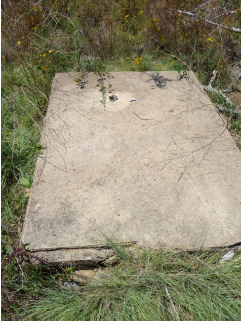
Image 7. Feature 3: Concrete Cistern
