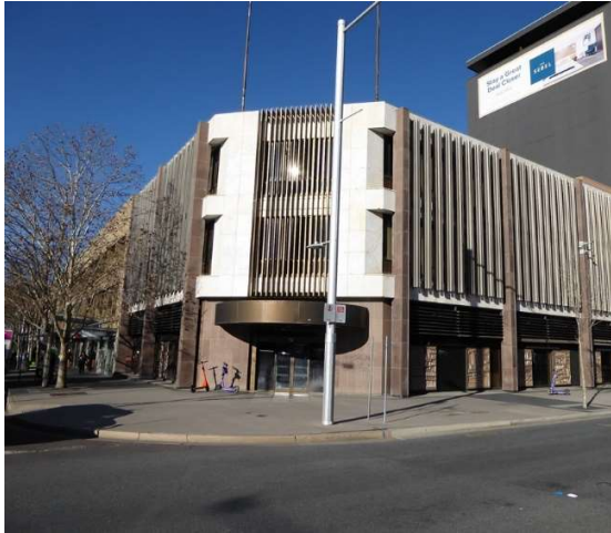
• Image 8: Former Commonwealth Bank Building from London Circuit.
