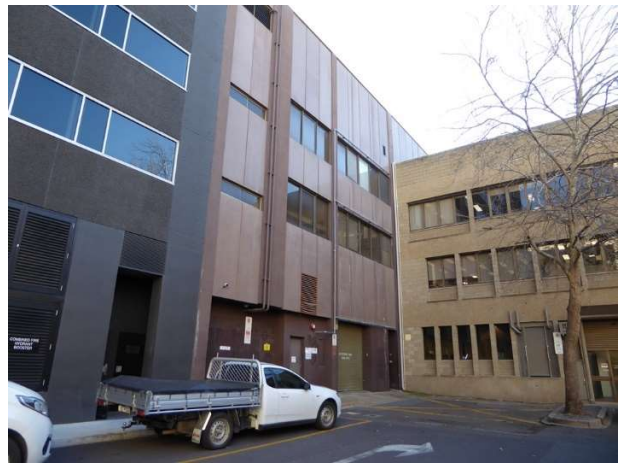
• Image 11: Former Commonwealth Bank Building rear elevation from Hillside Lane.
