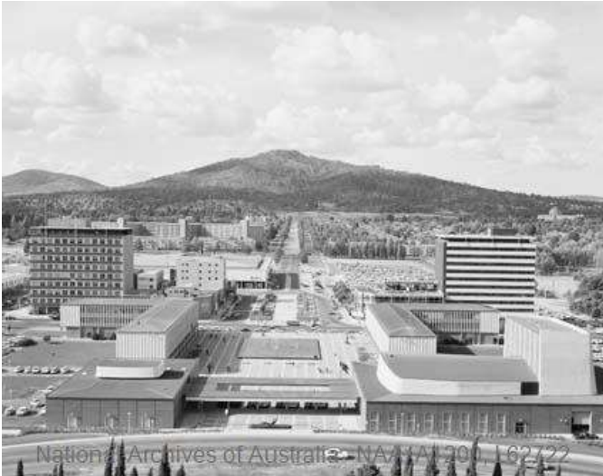
Figure 3: View along Ainslie Avenue towards Mount Ainslie in 1967 (NAA: A1200, L62722). Civic Square is located in the foreground and the FCBB is to the right in the middle distance.
