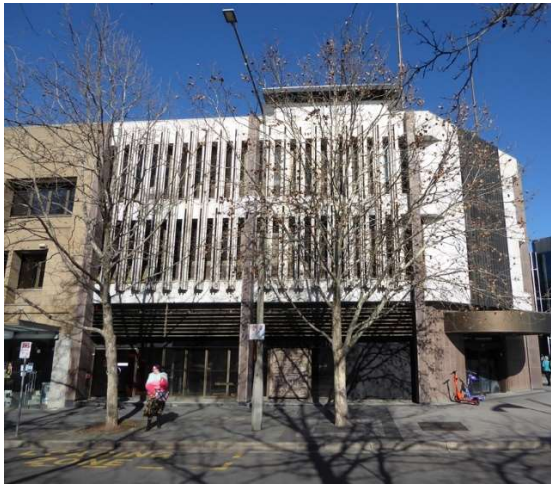
• Image 9: Former Commonwealth Bank Building from Ainslie Place.
