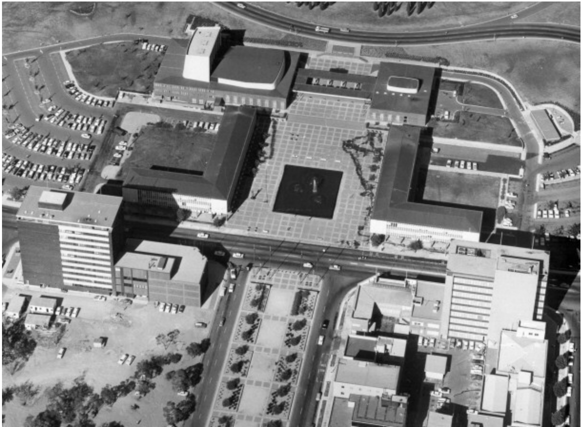
Image 2: Aerial view of Civic Square and Ainslie Avenue with the Former Commonwealth Bank Building centre left, late 1960s (ACT Heritage Library, Reference No. 000936).
