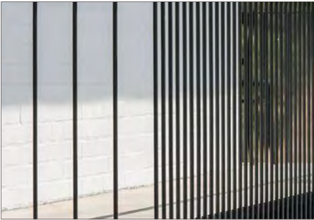
Balustrades disrupted the horizontal rhythm
