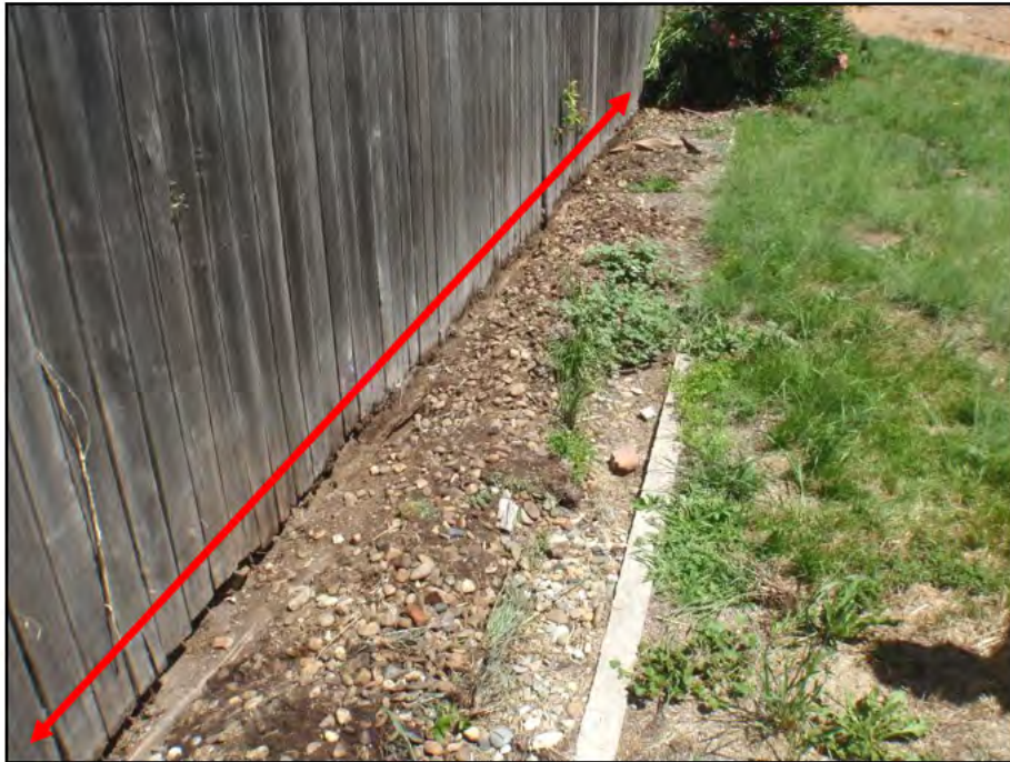
Photograph 1: Eastern boundary fence line garden bed of the 56 Belconnen Way block after removal of asbestos containing sheet debris
