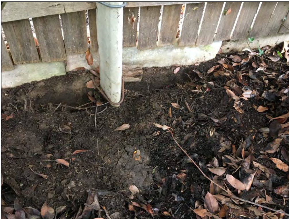
Area adjacent to the north property boundary after removal works
