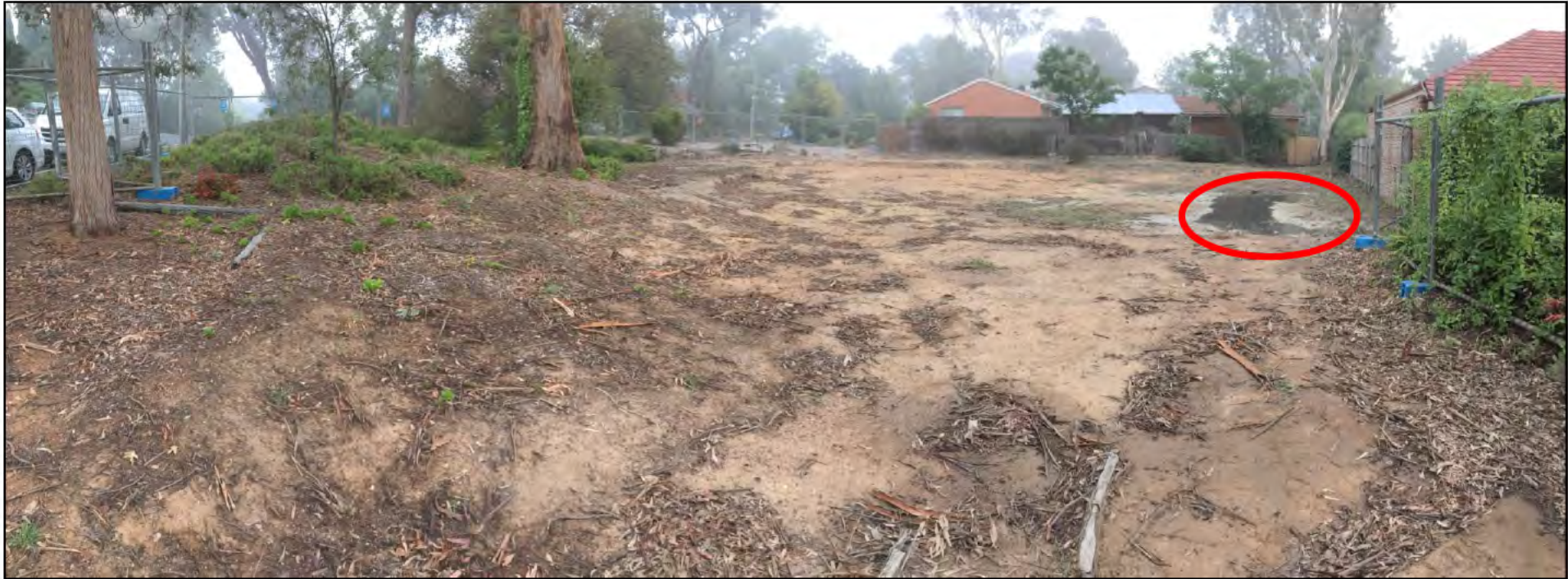
Entire block from northeast corner after removal works
