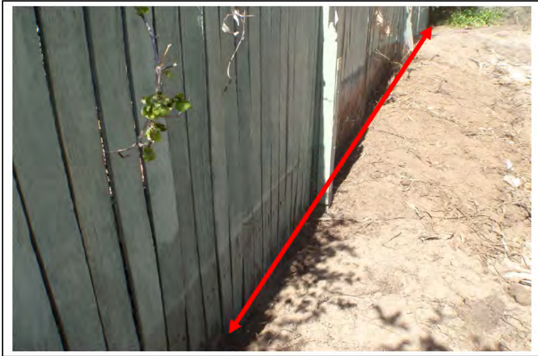
Photograph 1: Removal of non friable asbestos sheeting buried in the garden beds and along the southern boundary fence.
