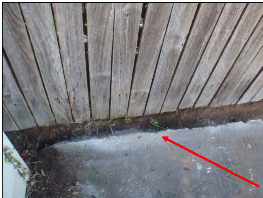
Photograph 2: Close up of edge of the concrete driveway section on the eastern boundary fence line from which ACM sheet was removed
