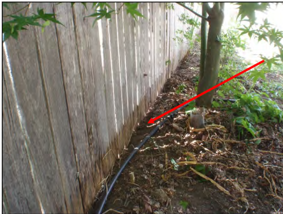
Photograph 4: Close up of northern side boundary fence line and garden bed from which ACM sheet and debris was removed
