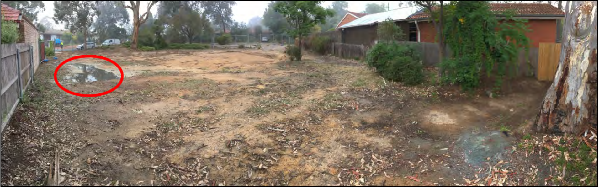
Entire block from northeast corner after removal works
