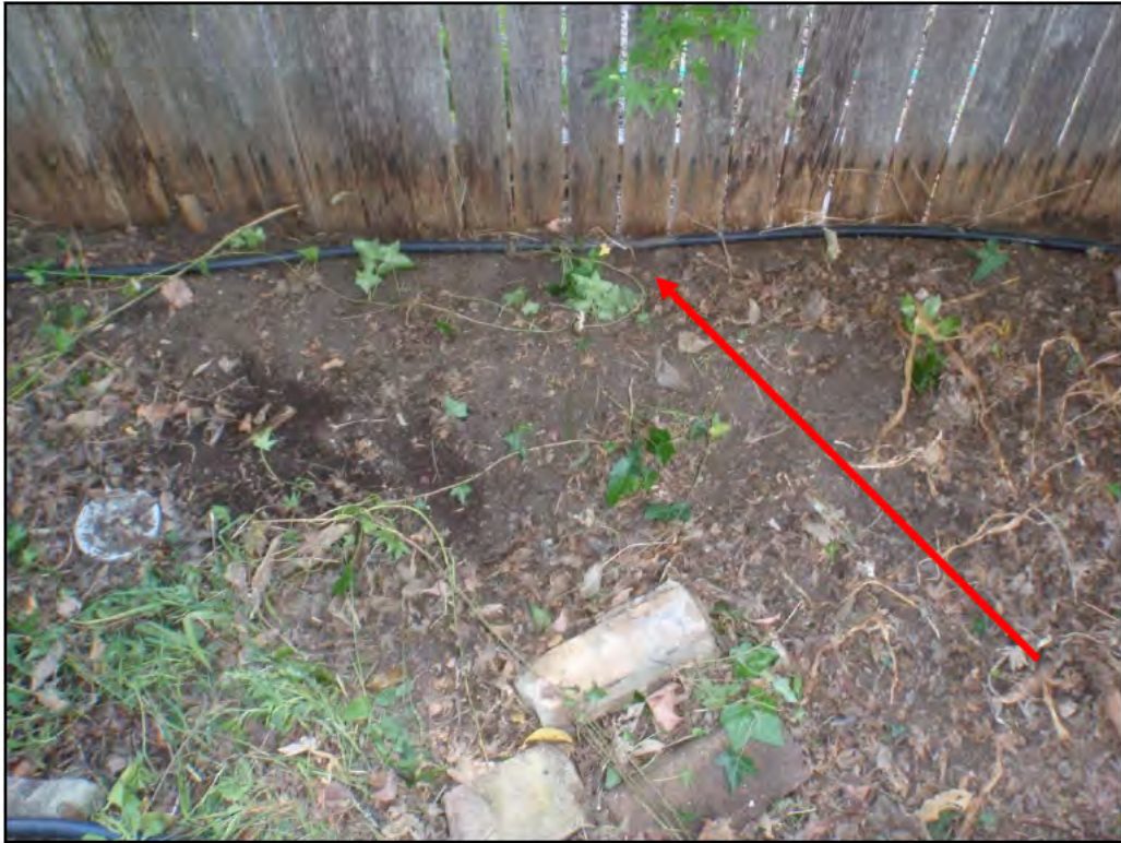
Photograph 5: Close up of northern side boundary fence line and garden bed from which ACM sheet and debris was removed
