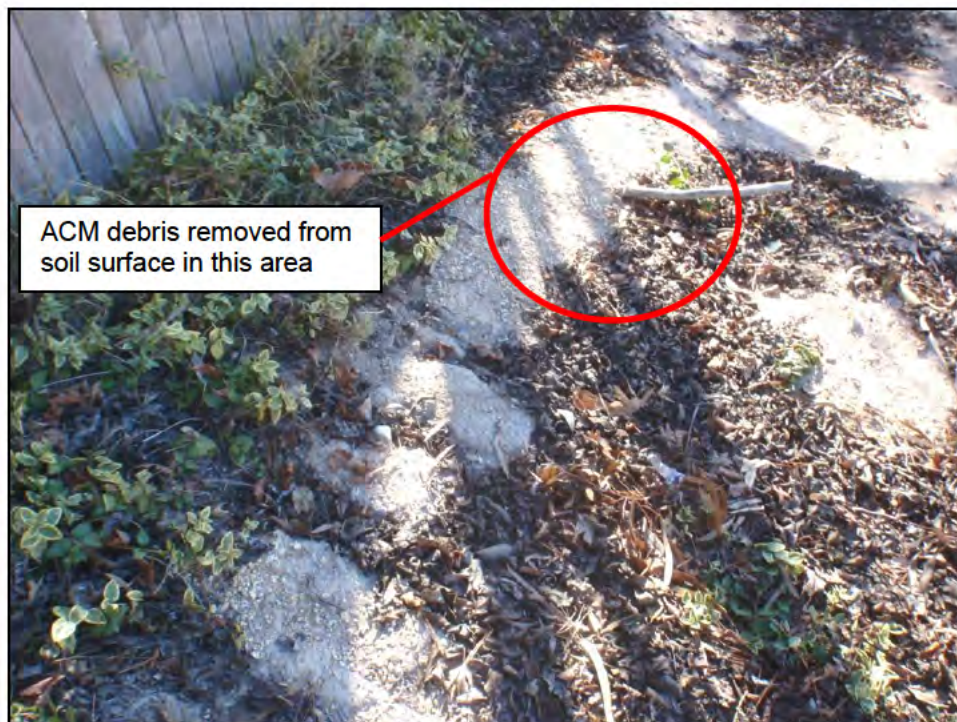
Photograph 4: 18 Darke Street Torrens block after removal of asbestos containing sheet debris located on top of the soil on the western side of the block
