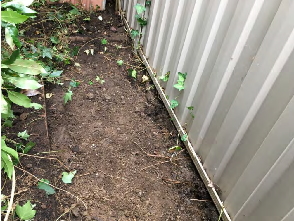
Area adjacent to the west property boundary after removal works
