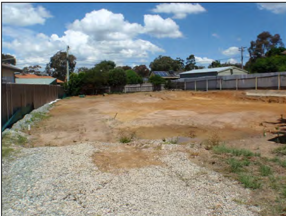
Photograph 4: 37 Rich St Higgins block after removal of asbestos containing sheet debris scattered in various locations across the top of the soil
