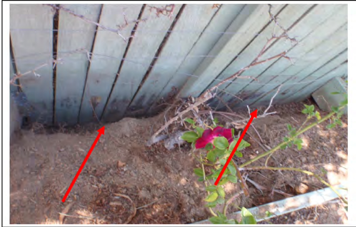
Photograph 3: Removal of non friable asbestos sheeting buried in the garden beds and along the southern boundary fence.
