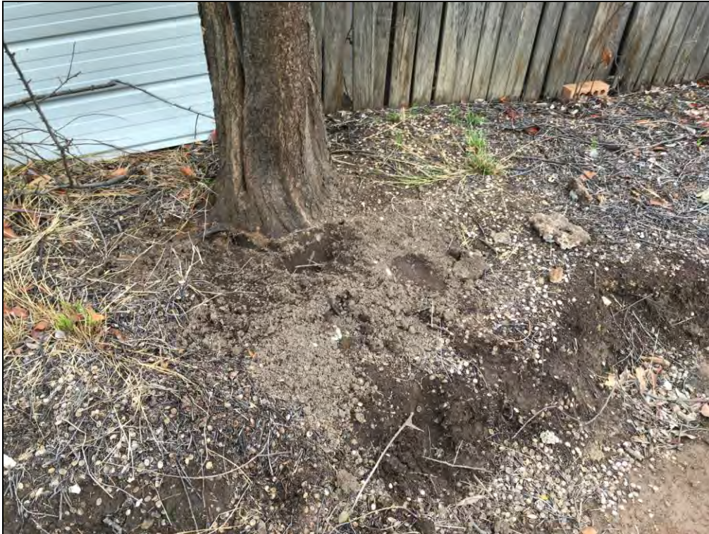
Area adjacent to the tree on the east property boundary after removal works
