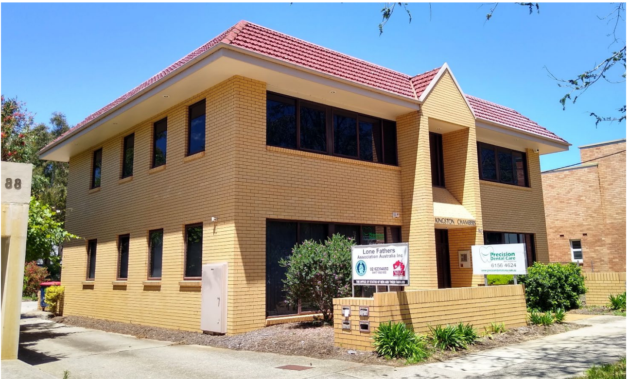
Figure 7 Kingston Chambers front and north side facade oblique angle (ACT Heritage 2020)
