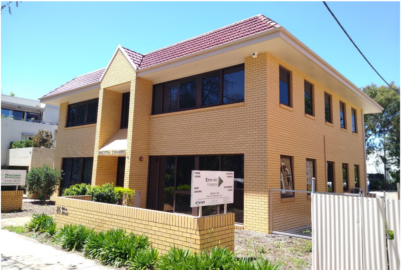
Figure 8 Kingston Chambers front and south side facade oblique angle (ACT Heritage 2020)
