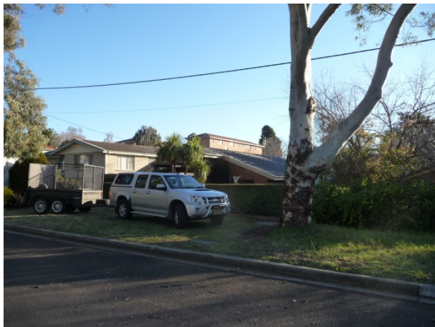
Figure 90 27 William Street - Block 28 Section 11 (ACT Heritage, 2014).
