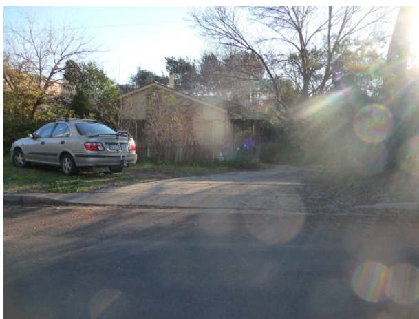
Figure 91 29 William Street - Block 29 Section 11 (ACT Heritage, 2014).
