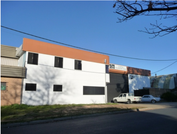
Figure 74 8-10 McEwan Avenue - Block 3 Section 8 (ACT Heritage, 2014).
