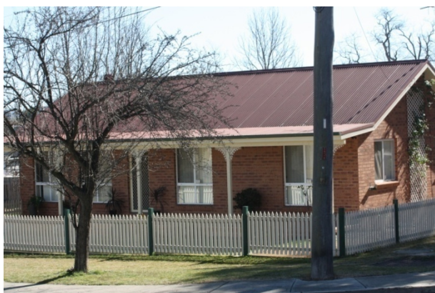
Figure 59 8 Hazel Street - Block 21 Section 8 (ACT Heritage, 2014).
