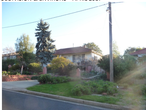
Figure 87 21 William Street - Block 25 Section 11 (ACT Heritage, 2014).
