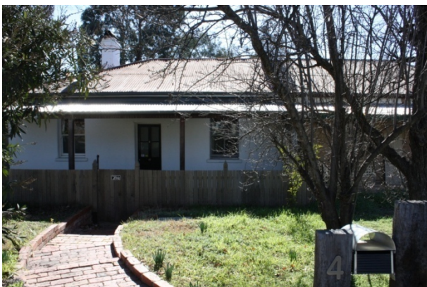
Figure 76 2 Hazel Street - Block 1 Section 11 (ACT Heritage, 2014).
