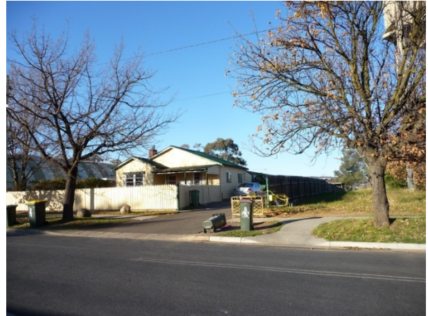
Figure 75 2 McEwan Avenue - Block 5 Section 10 (ACT Heritage, 2014).
