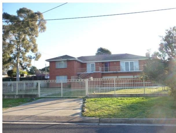
Figure 95 13-15 William Street - Block 37 Section 11 (ACT Heritage, 2014).
