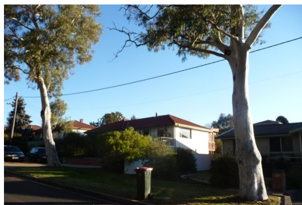
Figure 88 23 William Street - Block 26 Section 11 (ACT Heritage, 2014).
