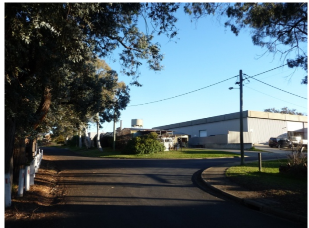
Figure 73 7 William Street/1 Hazel Street - Block 2 Section 10 (ACT Heritage, 2014).
