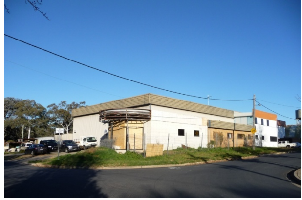
Figure 113 McEwan Avenue facing south (ACT Heritage, 2014).
