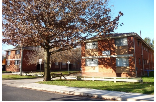
Figure 81 20-22 George Street - Carla Court - Blocks 10-11 section 11 (ACT Heritage, 2014).
