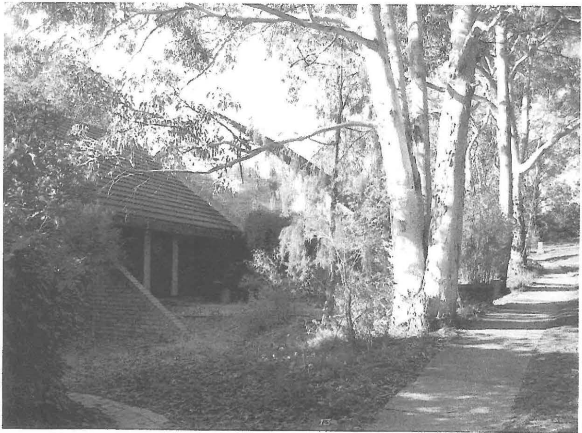
Figure 4: View from the access path to typical dwellings. Note the entry courtyard and mature landscape. DD 2004.
