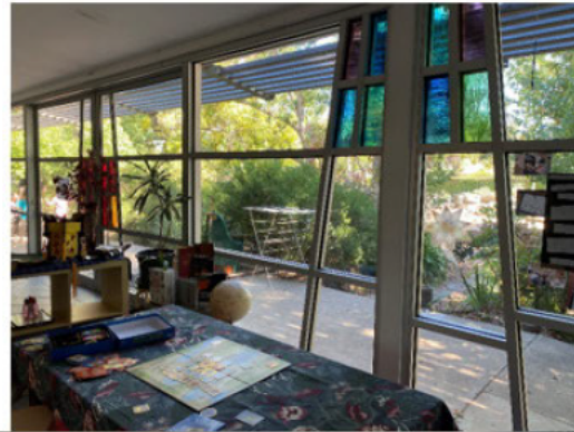
After Verandah Renovation
