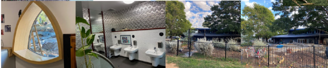
After Preschool Renovation
