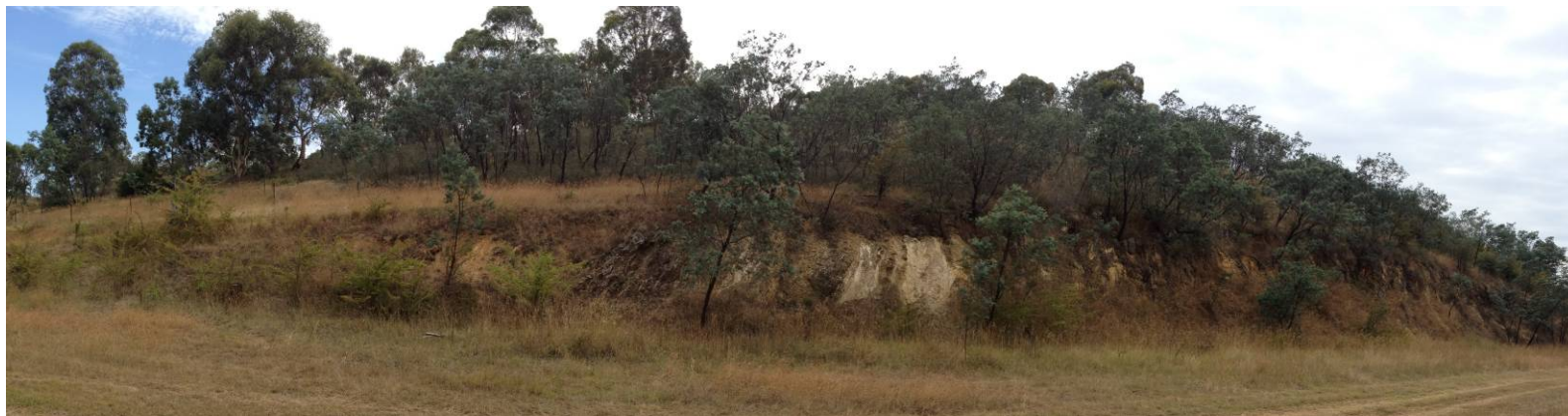
Figure 2 Barton Highway Road Cut, facing east towards Percival Hill. (ACT Heritage, 2017)
