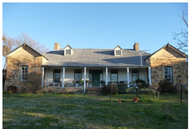
Figure 8 The Oaks north facade (ACT Heritage, 2014)
