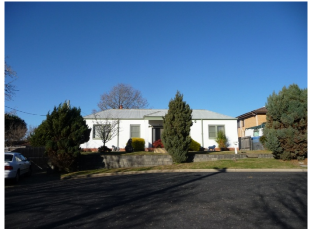
Figure 33 20 Florence St - Block 6 Section 6 (ACT Heritage, 2014).
