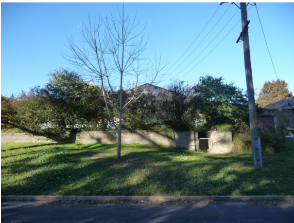
Figure 31 16 Florence St - Block 4 Section 6 (ACT Heritage, 2014).
