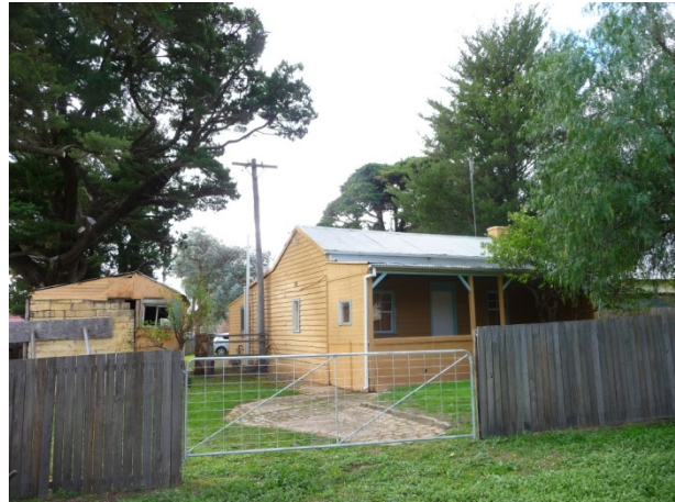
Figure 9 Robertsons House south facade (ACT Heritage, 2014)
