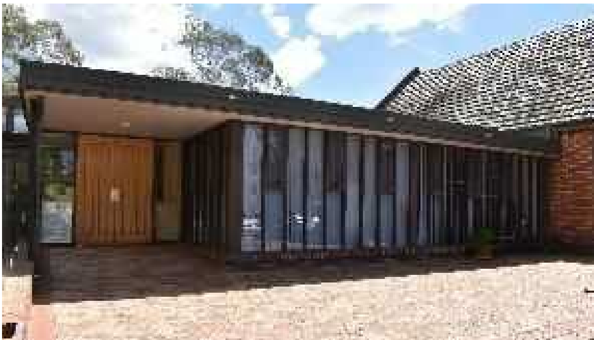
Figure 11 - Exterior photo of extension building in 2020 (Hyperspace 2020)
