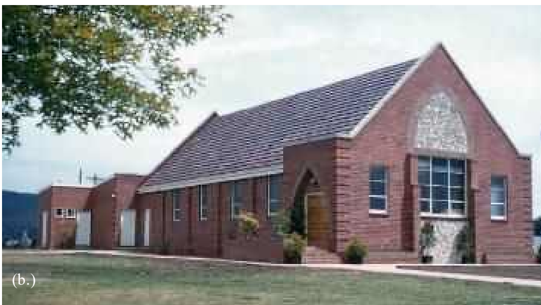
Figure 2 - The hall, which was used as the original church building: (a.) Plans for the constructed portions of the church hall and welfare room (ACTPLA in Hyperspace 2020); (b.) The hall before the development of the church was completed in 1971 (Chad Clarke, Canberra National SDA, in Hyperspace 2020).
