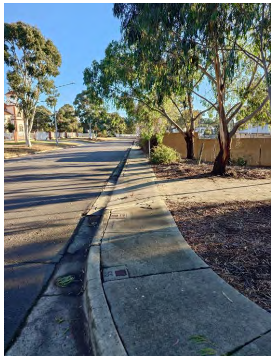
Figure 90 – Footpath in Northern Verge of Georgina Crescent (south)
