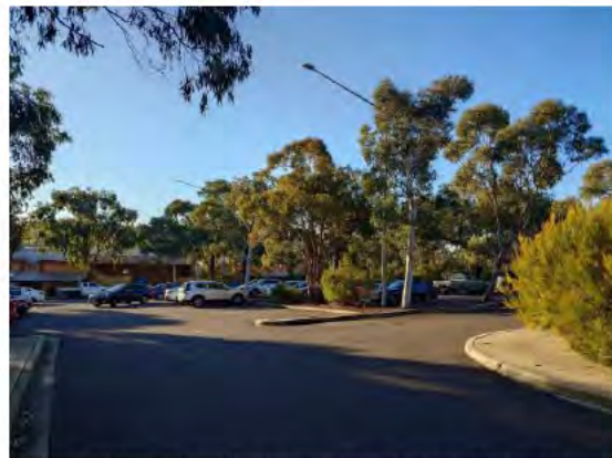
Figure 47 – Streetlights in Southern Car Park
