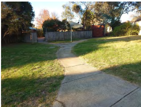
Figure 88 – Footpaths Branching East into Residential Developments in Section 28 Kaleen
