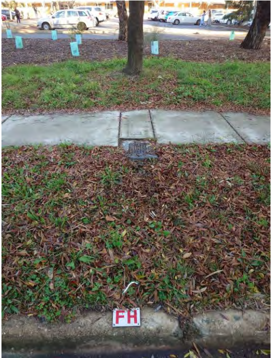
Figure 20 – Existing Fire Hydrant in Maribyrnong Avenue
