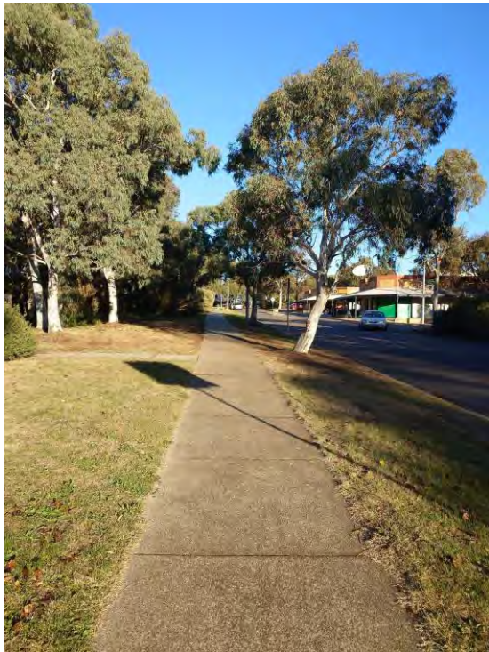
Figure 87 – Footpath in West Verge of Georgina Crescent (east)
