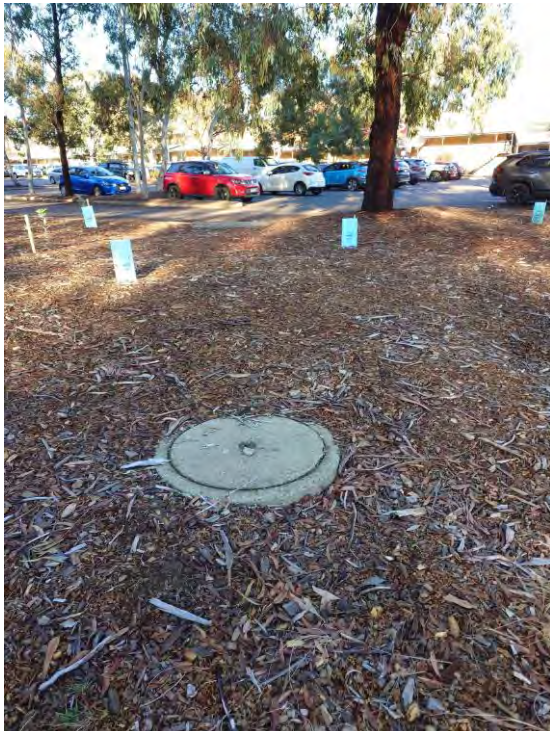
Figure 11 – Sewer Manhole in North West Corner of Site
