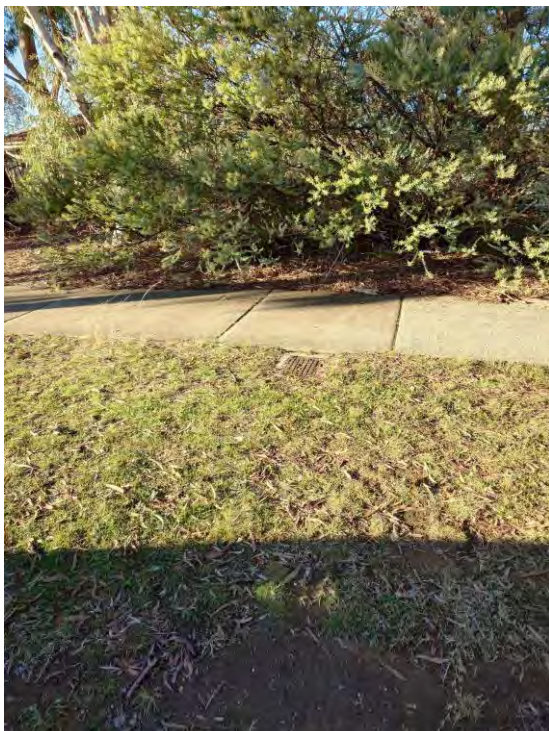
Figure 23 – Existing Fire Hydrant in Georgina Crescent (east)
