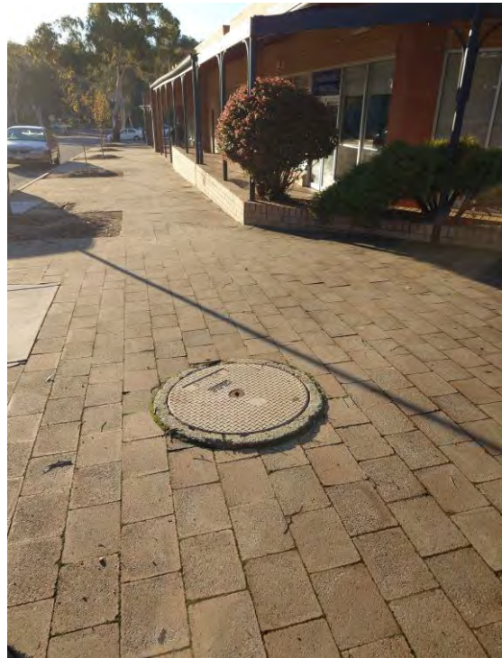
Figure 14 – Sewer Manhole over Main Extension through Northern Internal Road from Georgina Crescent (west)
