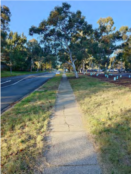
Figure 83 – Footpath in Northern Verge of Maribyrnong Avenue
