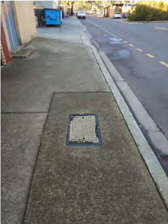
Figure 36 – Telstra Pit in Southern Internal Access Road
