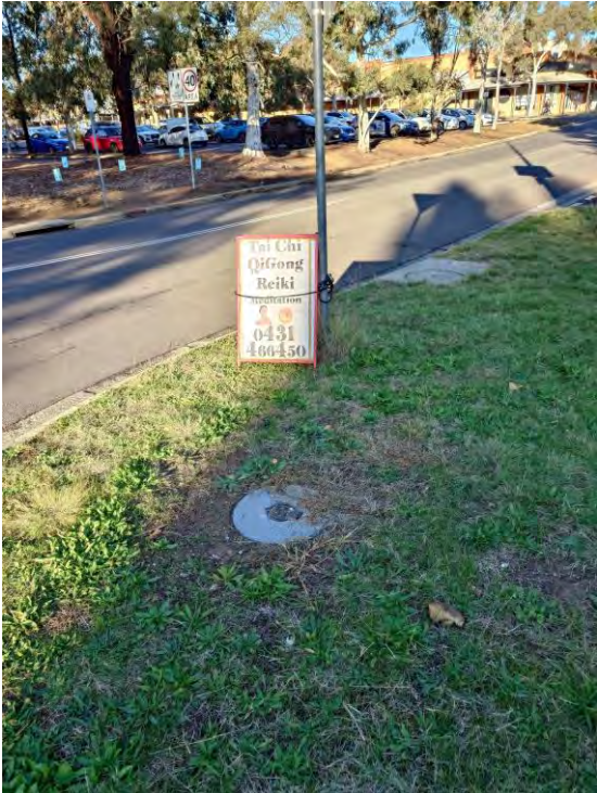
Figure 18 – Stop Valve over DN150 Water Main at Intersection of Maribyrnong Avenue and Georgina Crescent (west)
