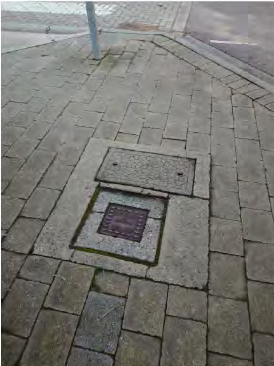
Figure 34 – Telstra Pit in Southern Internal Access Road
