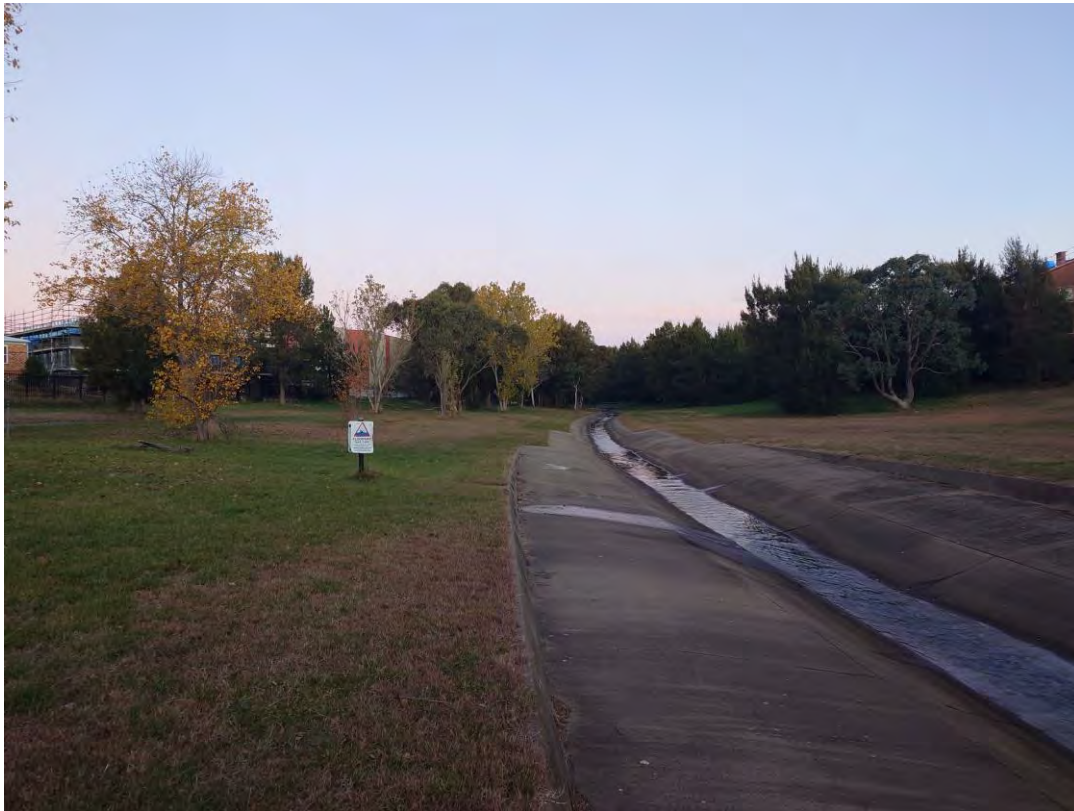
Figure 32 – Concrete Lined Channel in Baldwin Drive Looking South
