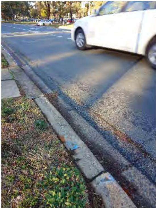
Figure 55 – Kerb Survey Marker on Maribyrnong Avenue
