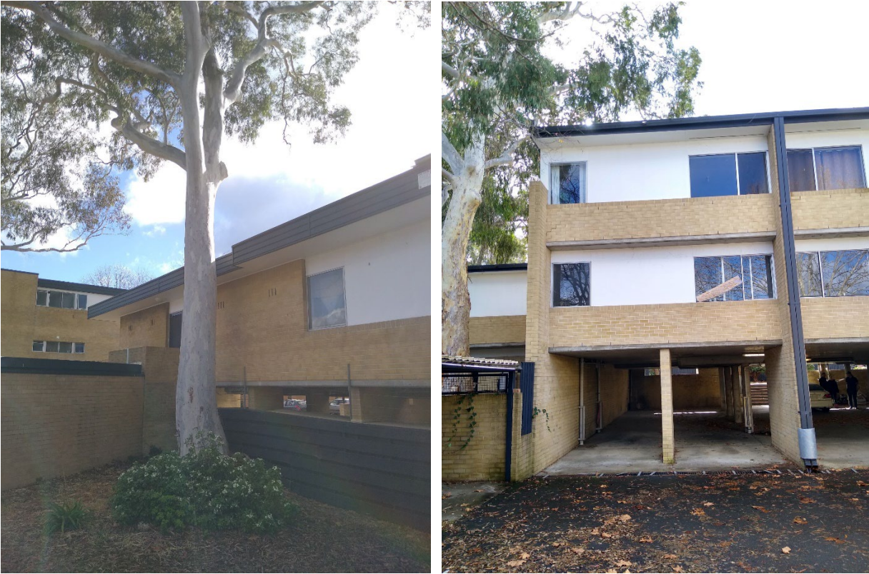
Figure 7 Jerilderie Court - Units 13-14 tree allowances in roof design; Figure 8 Jerilderie Court - Units 32-35 undercroft parking external
