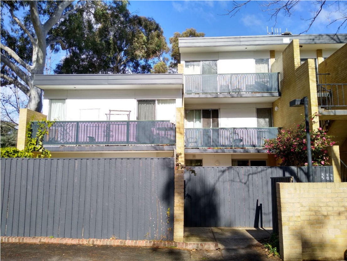
Figure 5 Jerilderie Court - units 1 2 4 6
