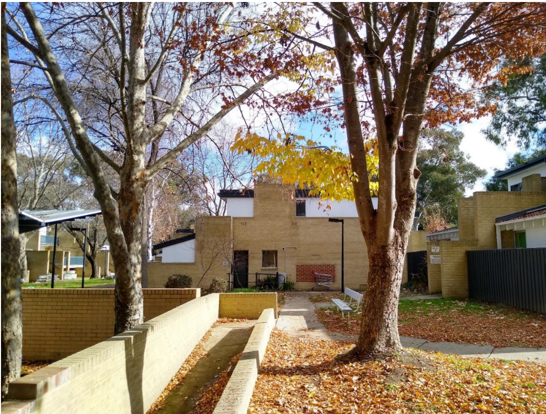
Figure 2 Jerilderie Court - Common area central facing west
