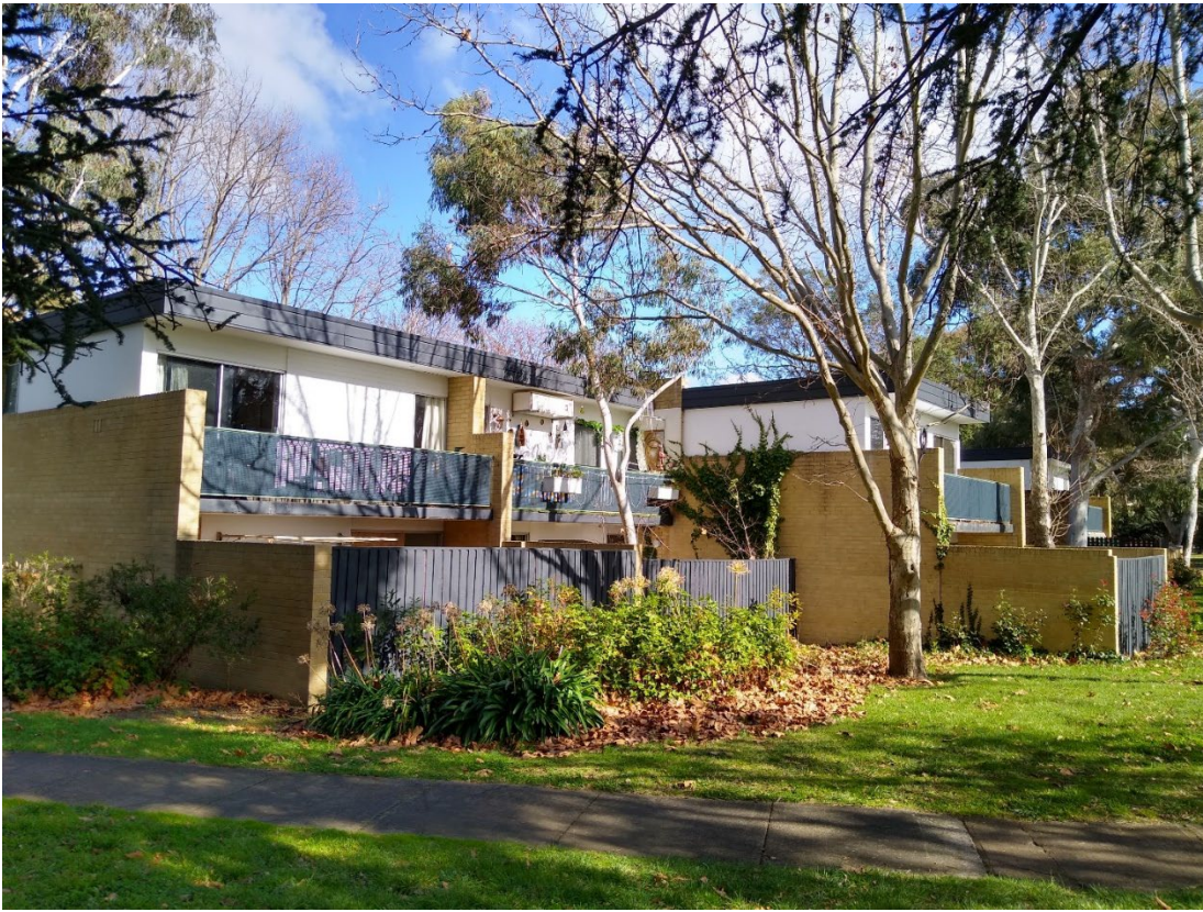
Figure 1 Jerilderie Court - northeast corner facing southwest
