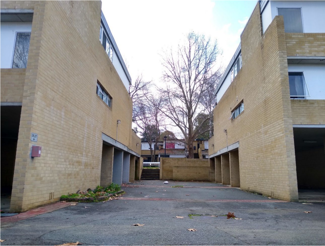
Figure 3 Jerilderie Court – internal car access and mews parking facing central area with units 28-31 left and 21-25 right
