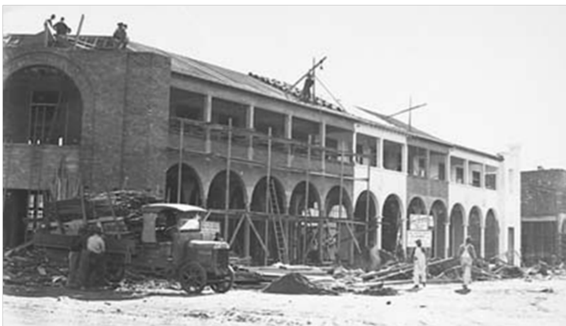
The Melbourne Building under construction, mid-1920s.
