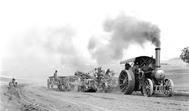
Image 4 One of the Fowler locomotives towing a New Era grader (Mildenhall Collection cited in Lamb 2015)
