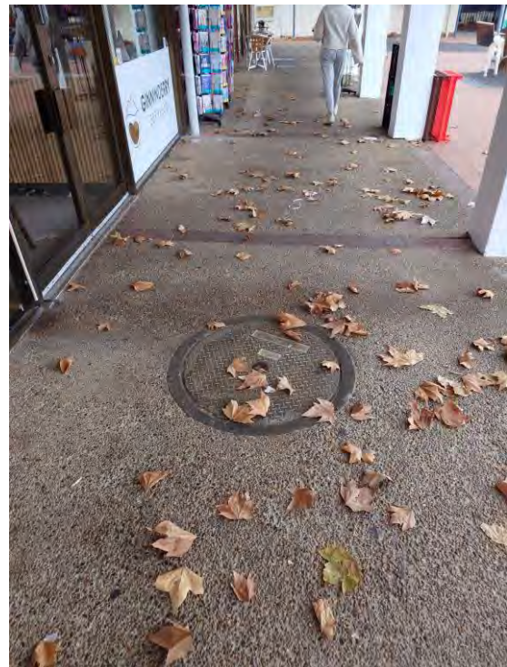
Figure 52 – Stormwater Manhole in Group Centre (central) Verge
