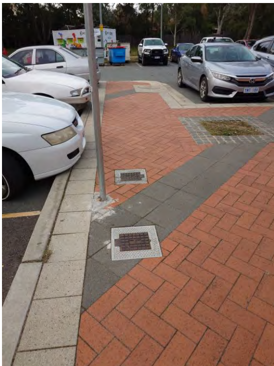
Figure 30 – Double Hydrants in Charnwood Place (west)
