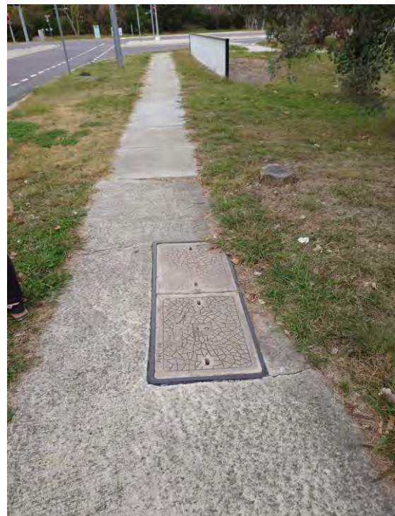
Figure 70 – Telstra Pit in Lhotsky Street South Verge
