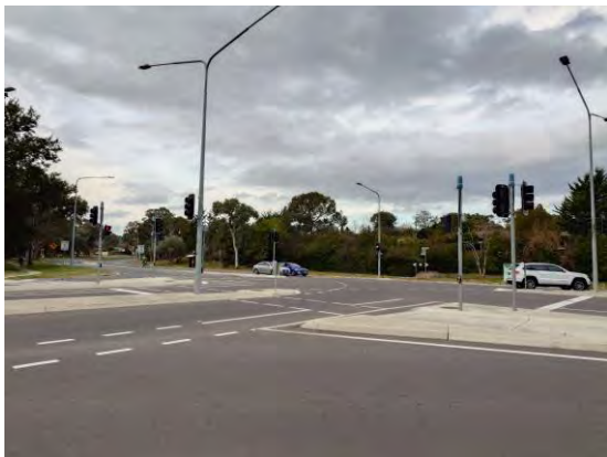
Figure 86 – TCCS Streetlights at Intersection of Lhotsky Street and Tillyard Drive
