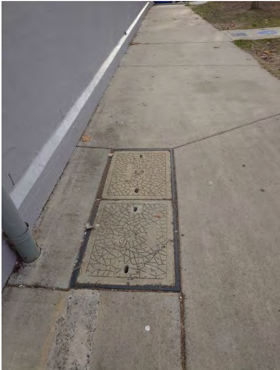
Figure 66 – Telstra Pit North of Site
