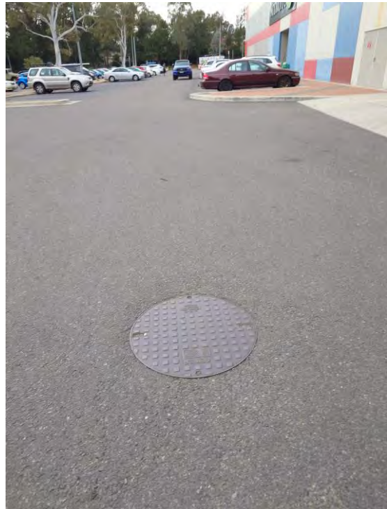
Figure 17 – Sewer Manhole over DN300 Main in Charnwood Place (west)
