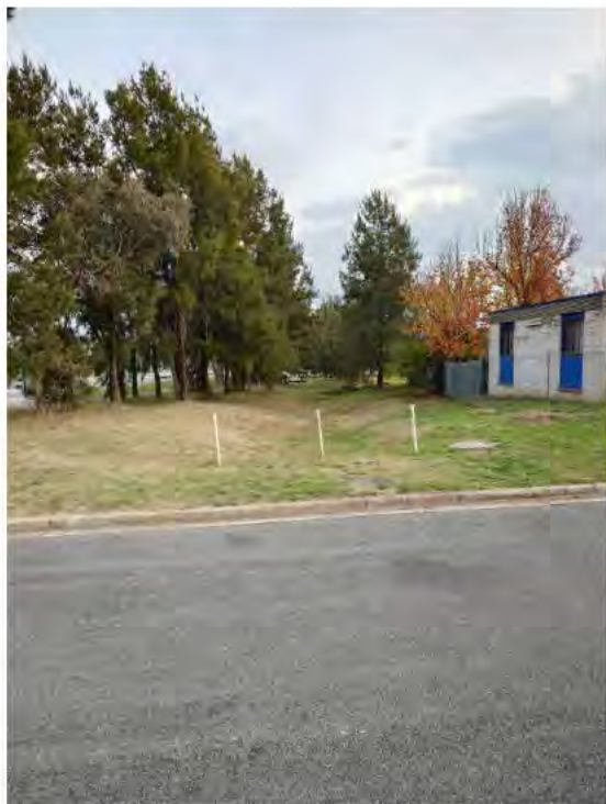
Figure 56 – Stormwater Swale through Block 29 Section 95 Looking South
