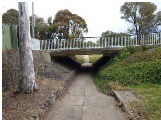
Figure 140 – Lhotsky Street Underpass
