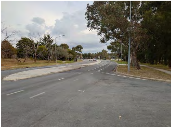
Figure 84 – TCCS Streetlights on Tillyard Drive
