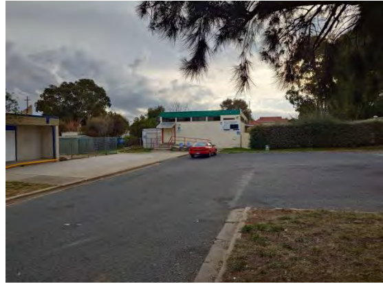
Figure 107 – General View of Verge Place
