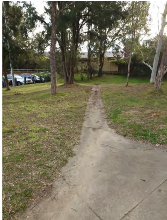
Figure 60 – Stormwater Swale and Concrete Invert North West of Site
