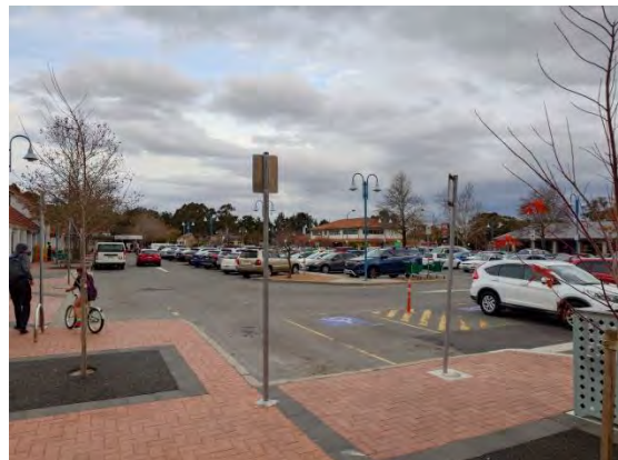
Figure 88 – TCCS Streetlights in Charnwood Place (east) Car Park
