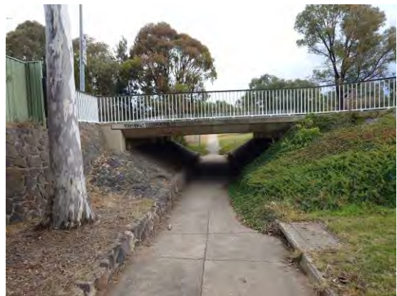
Figure 61 – Lhotsky Street Underpass South West of Site
