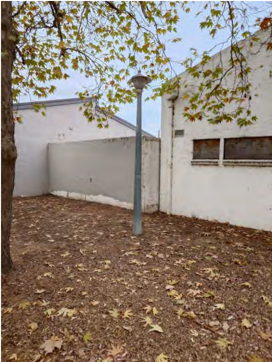
Figure 82 – TCCS Streetlight in South West Portion of Site (Block 46 Section 95)
