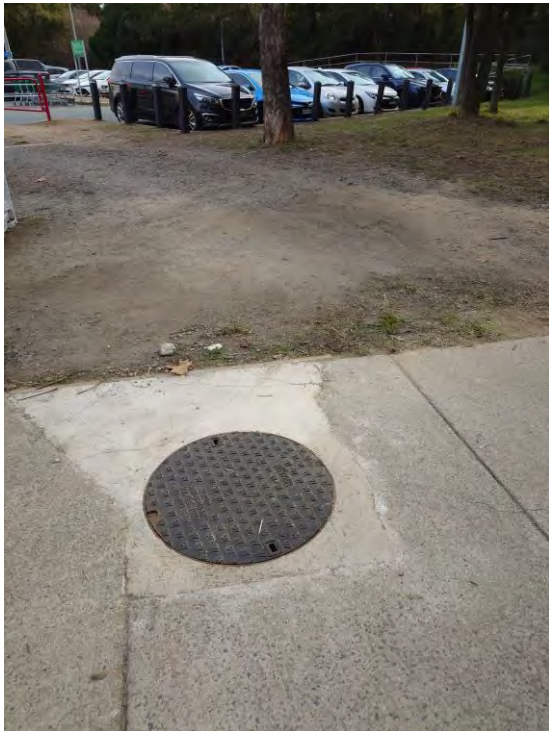
Figure 15 – Sewer Manhole over DN300 Main North of Charnwood Place (west)
