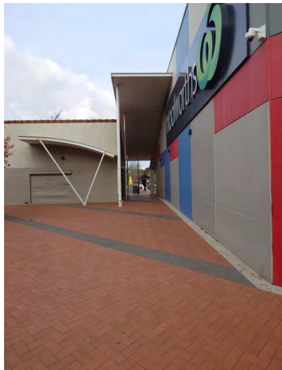
Figure 135 – Fully Paved Verge in Charnwood Place (west) Car Park
