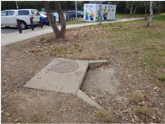
Figure 47 – Existing Stormwater Plantation Sump North West of Site
