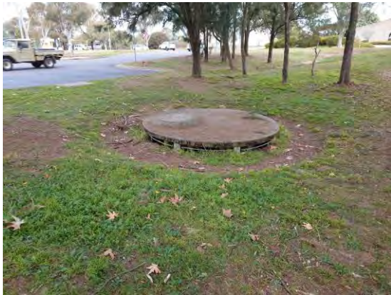
Figure 49 – Inlet/Surge Structure at Junction of DN1350 and DN1800 Pipes (west)
