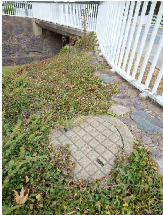
Figure 21 – Sewer Manhole at DN300 and DN525 Junction in Lhotsky Street
