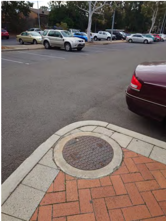
Figure 19 – Sewer Manhole over DN300 Main in Charnwood Place (west)
