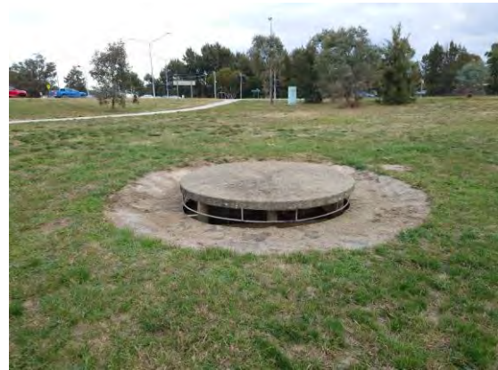
Figure 51 – Existing Stormwater Inlet/Surge Structure in Block 20 Section 97
