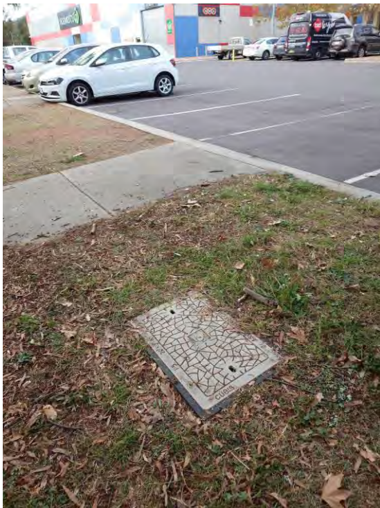
Figure 68 – Telstra Pit in Charnwood Place (west)
