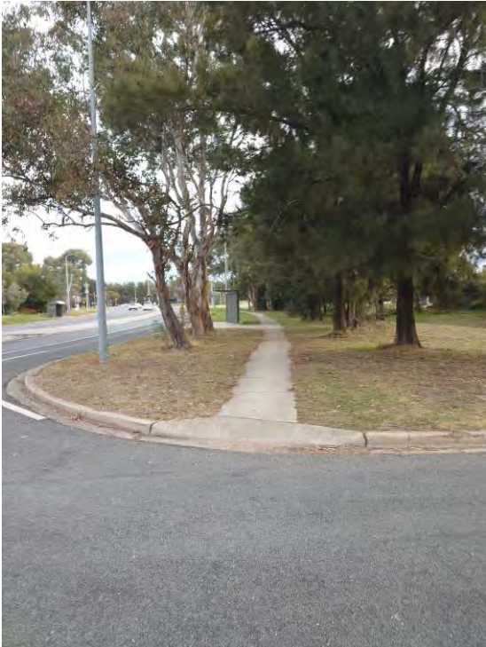
Figure 128 – Footpath in West Verge of Tillyard Drive
