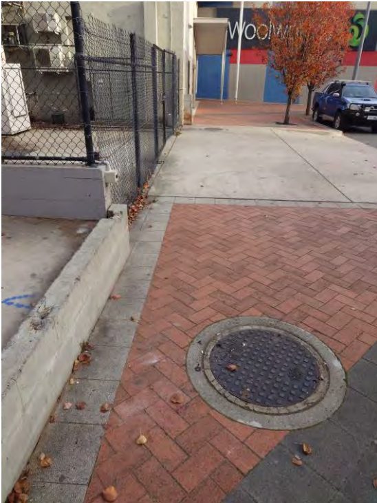
Figure 45 – Existing Stormwater Manhole in Charnwood Place (west) Verge
