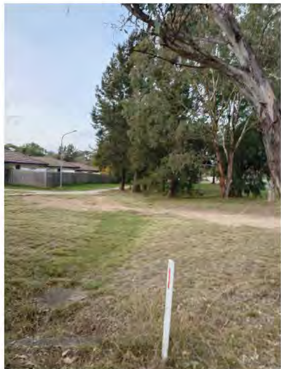
Figure 57 – Stormwater Swale and Plantation Sump North West of Site
