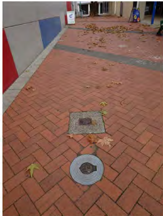
Figure 28 – Fire Hydrant and Stop Valve on DN150 Main Near Charwood Place (west)
