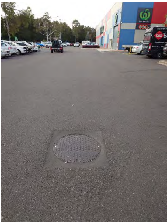
Figure 16 – Sewer Manhole over DN300 Main in Charnwood Place (west)
