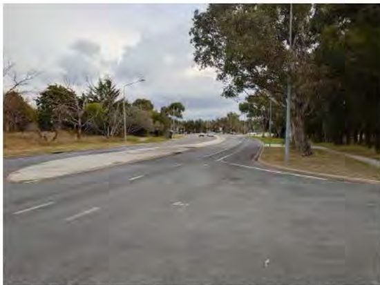
Figure 97 – General View of Tillyard Drive Looking South
