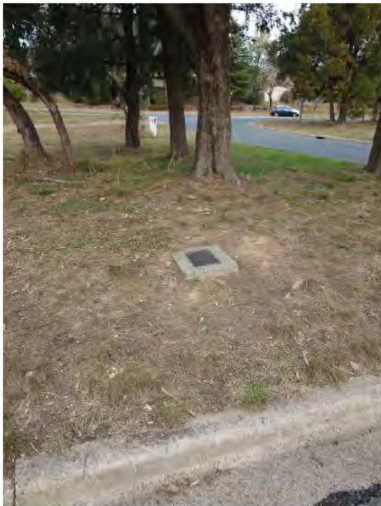
Figure 27 – Existing Fire Hydrant on Dead End DN150 in Verge Place
