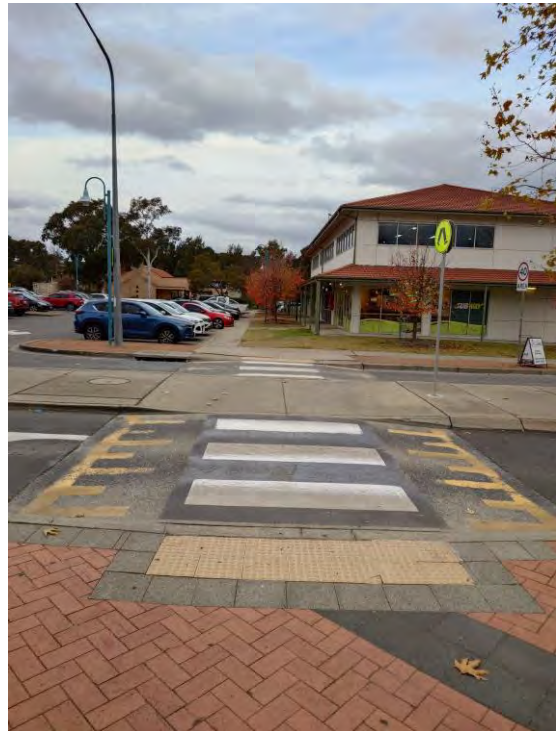
Figure 143 – Raised Pedestrian Crossing in Charnwood Place (east)
