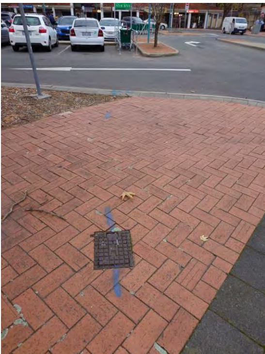
Figure 38 – Existing Fire Hydrant in Charnwood Place (east)
