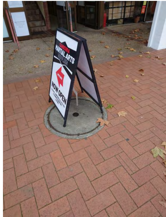
Figure 25 – Sewer Manhole in Group Centre (central)
