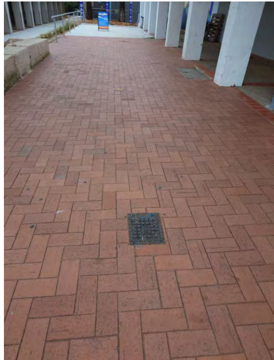
Figure 39 – Existing Fire Hydrant in Central Carpark (west)
