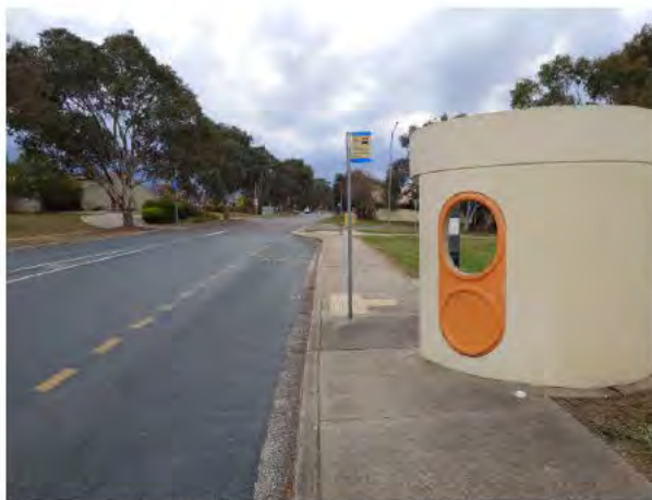
Figure 148 – Bus Stop on Lhotsky Street Near Charnwood Place (west)
