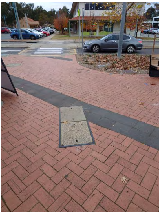
Figure 72 – Telstra Pit in South West Central Car Park
