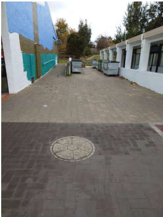
Figure 24 – Sewer Manhole in Group Centre (central)
