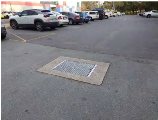
Figure 48 – Stormwater Grated Pit in West Car Park
