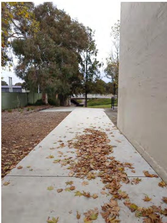
Figure 137 – Footpath Leading from Group Centre to Lhotsky Street Underpass
