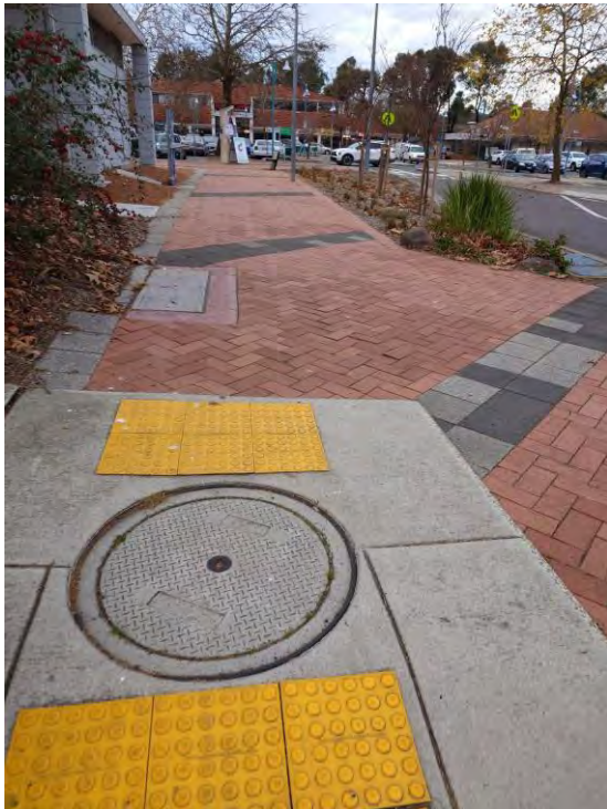
Figure 23 – Sewer Manhole in Group Centre (east)
