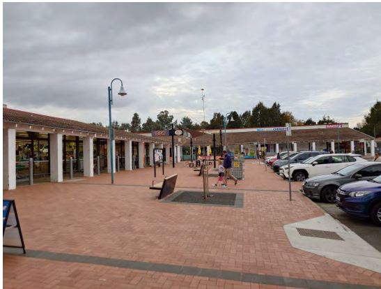
Figure 145 – General Photo of Fully Paved Verge in Group Centre
