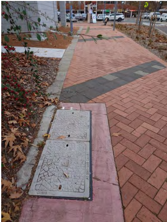
Figure 71 – Telstra Pit in Charnwood Place (east) West Verge
