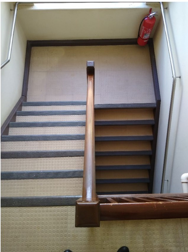
Figure 11: Internal staircase and timber banister
