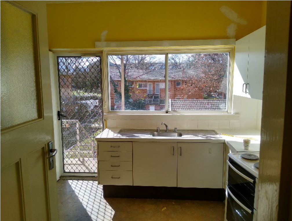
Figure 12: Renovated kitchen area of an apartment
