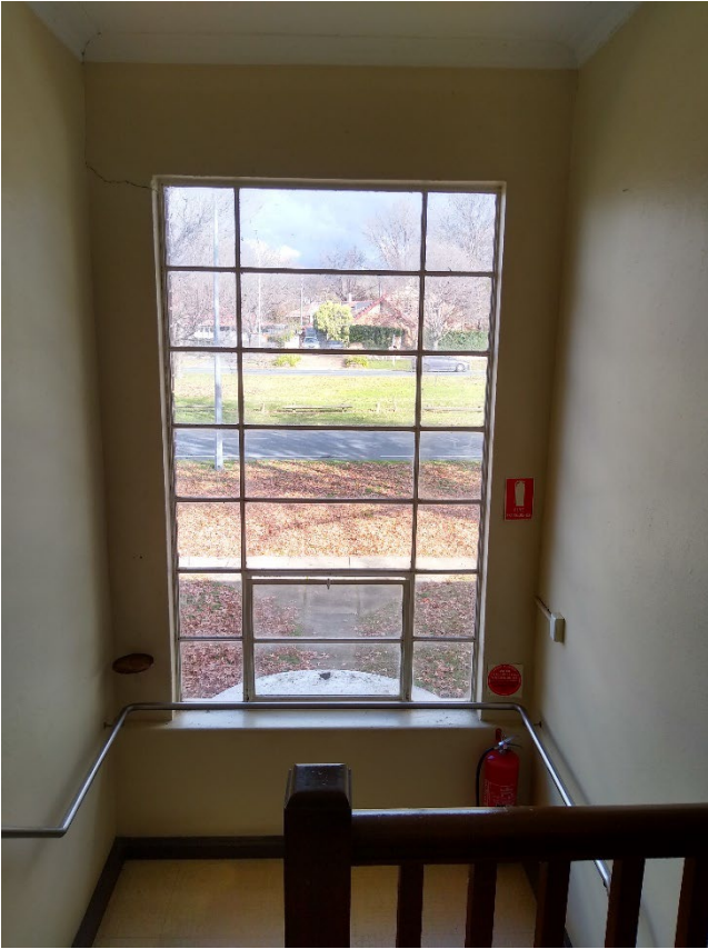
Figure 10: Original internal staircase, banister and windows with street view
