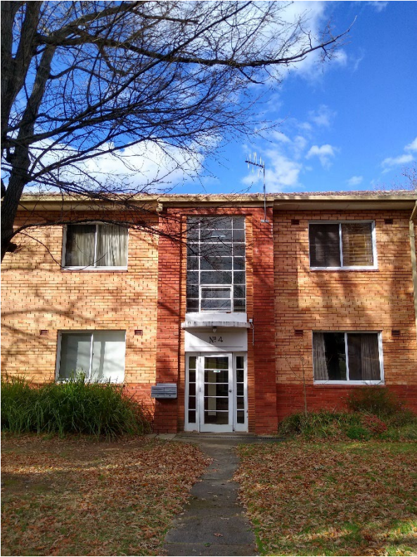
Figure 4 No.4 Building entrance.
