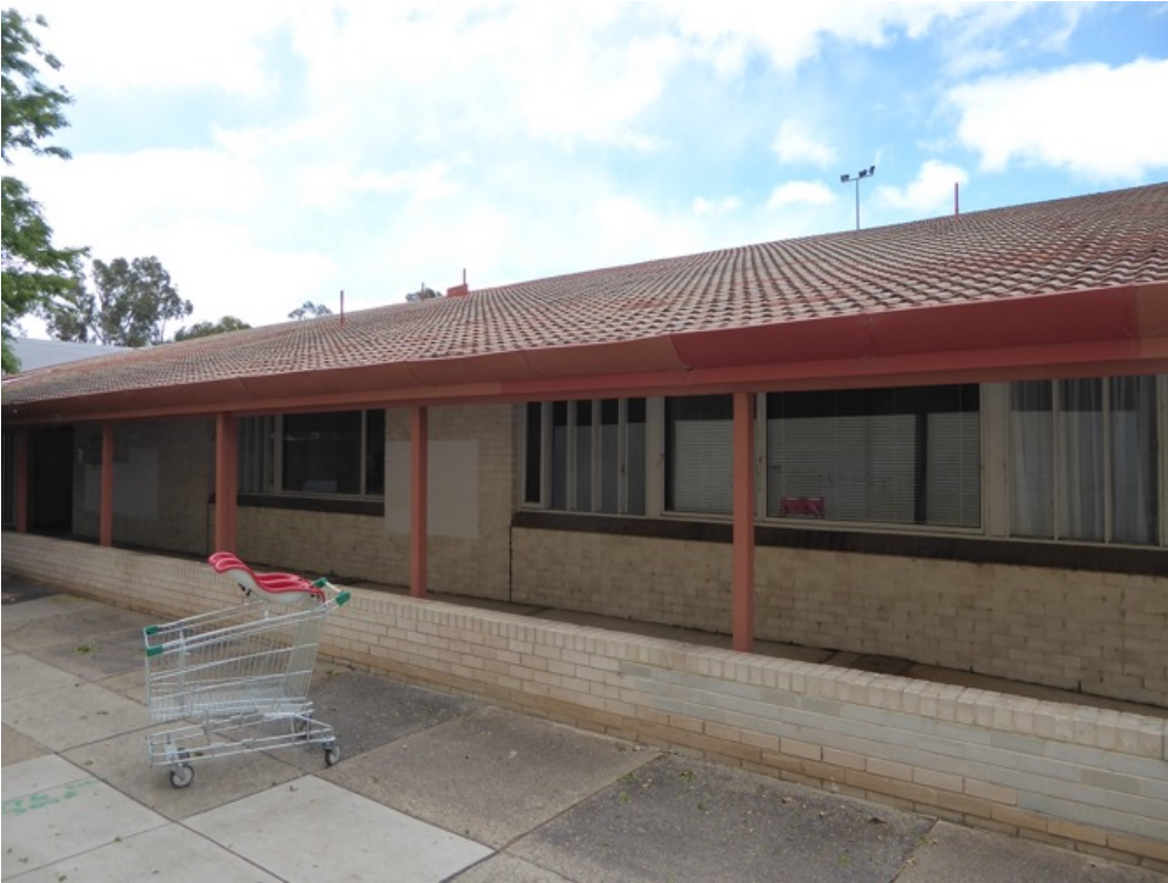
Figure 12 View of southwest side of the Centre with verandah
