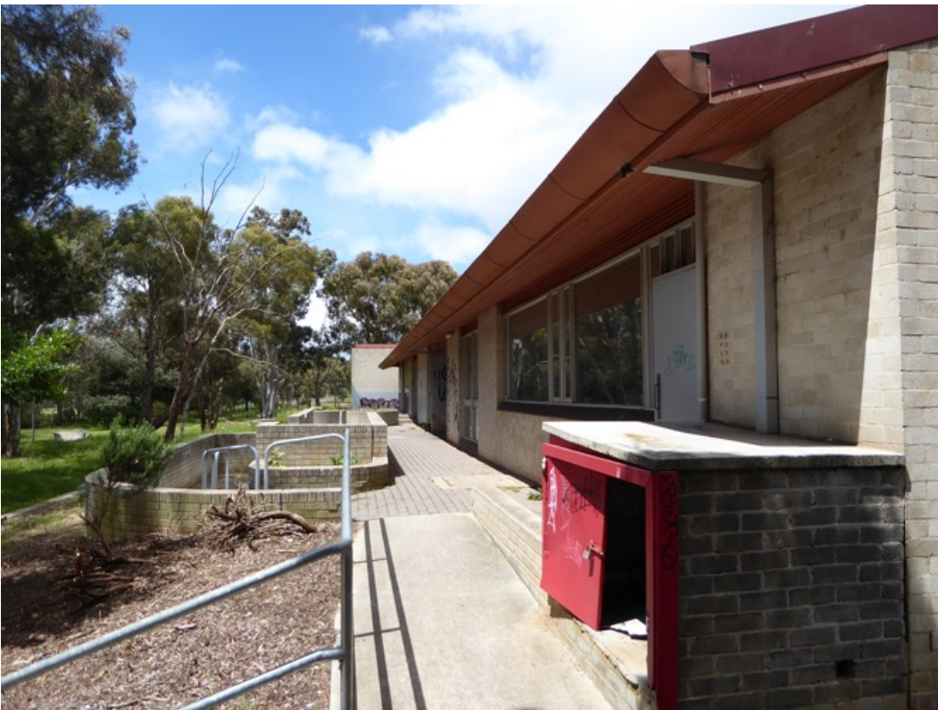
Figure 13 View of the northwest side of the Centre
