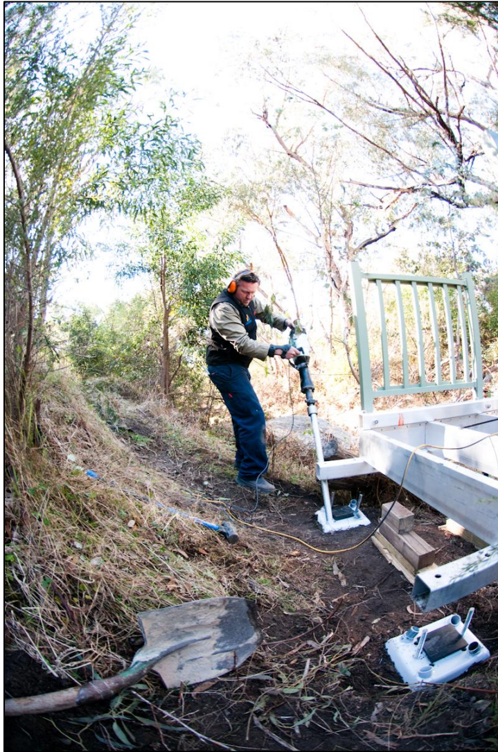
Figure 1.4 Installation of platform
