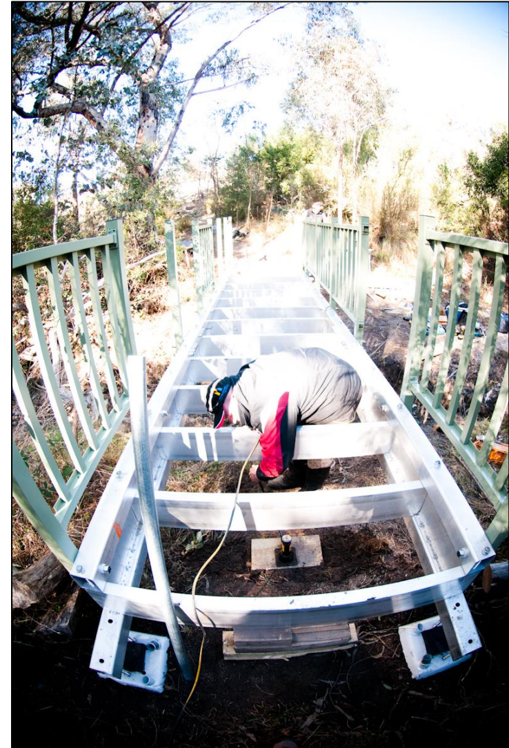
Figure 1.5 Installation of platform
