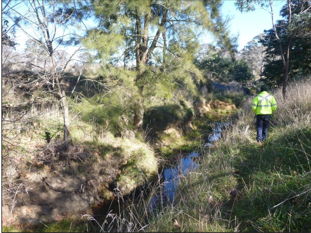
Figure 3.1 View west along Halls Creek showing gullying and erosion of the creek to bedrock
