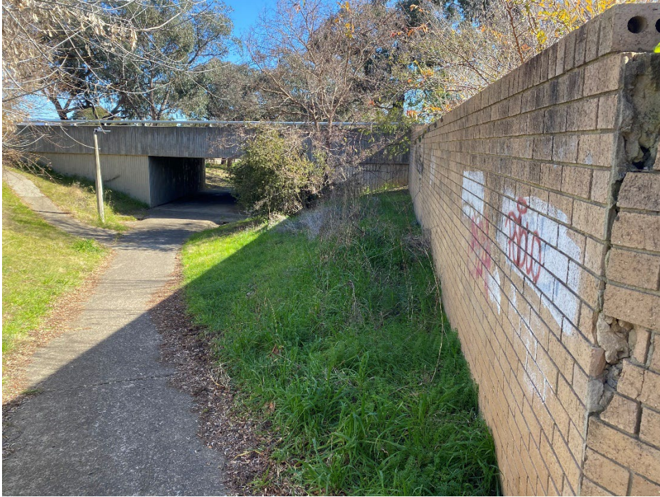
Southern boundary of site (facing west)
