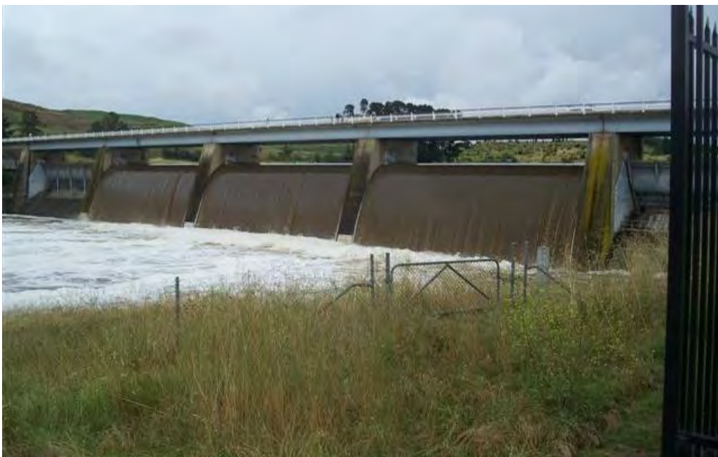
Scrivener Dam – three floodgates open following heavy rain in December 2010
