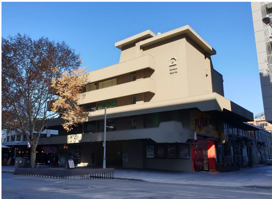
Image 1. Cinema Center from Buda Street, (ACT Heritage, 2019)
