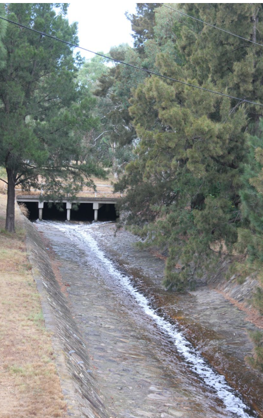
ARMoured CHANNEL, STREETON DRIVE
