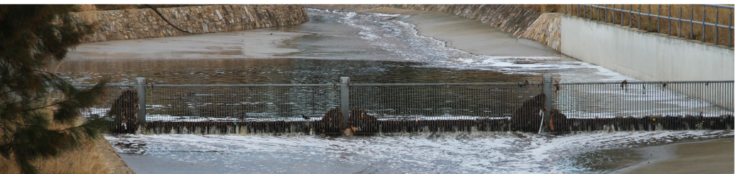
TRASH RACK AND LINED CHANNEL, DIXON DRIVE
