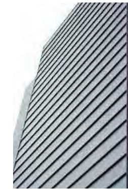
BALCONY CLADDING - TOWER
