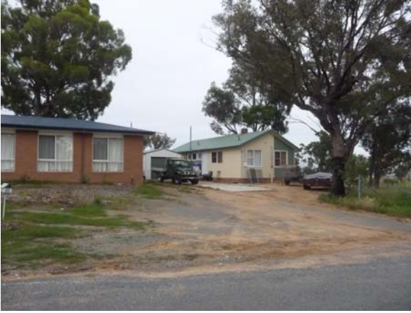
Cottage 1 on RHS
