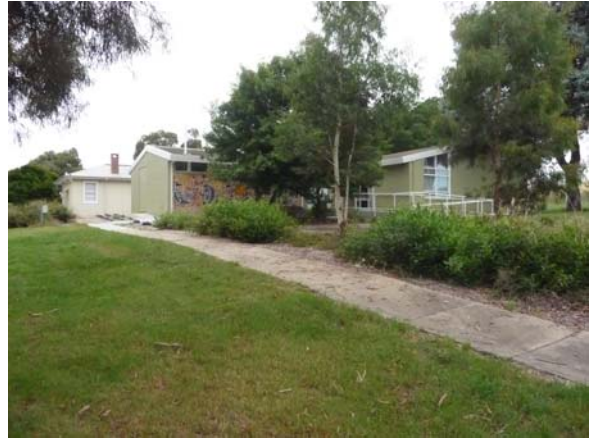
1969 school building to front. 1937 school building behind
