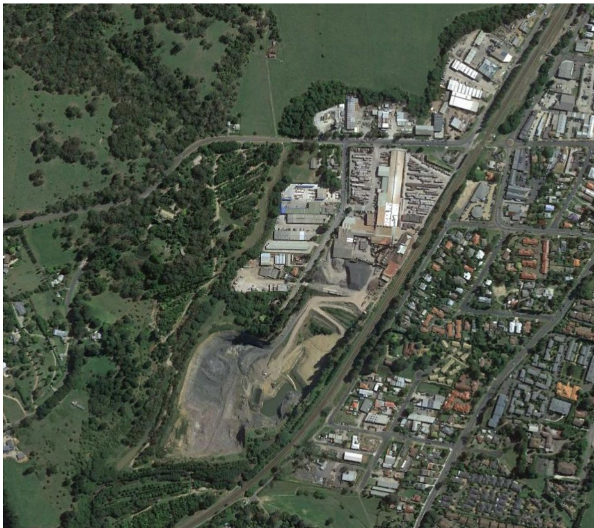
Figure 2.35 Aerial view of Bowral Bricks. (Source: Google Earth, 2017)
