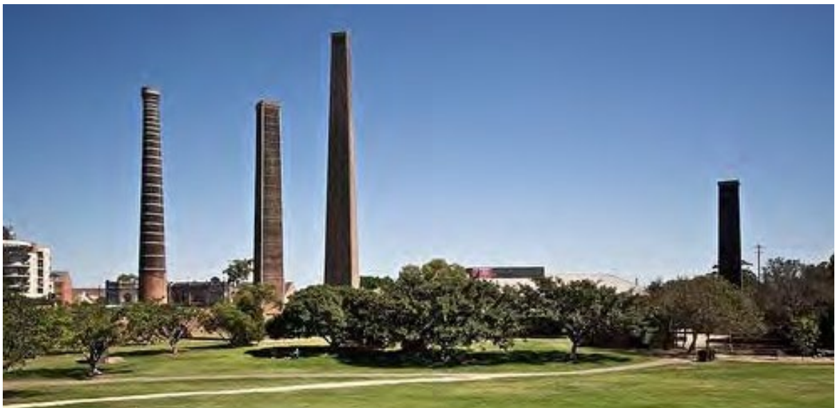
Figure 2.28 Stacks at the former Bedford Brick Works, with Sydney Park in the foreground, 2008. (Source: Flickr)
