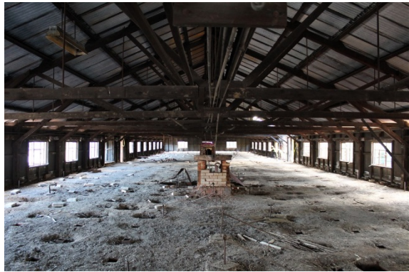
Figure 3.8 Upper firing floor of Hardy Patent Kiln 2 (Element 5). (Source: GML, 2017)
