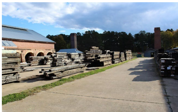
Figure 3.38 First brickyard (Element 37), looking west. (Source: GML, 2017)
