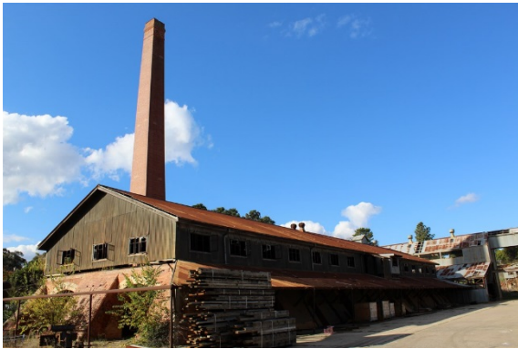
Figure 3.7 Hardy Patent Kiln 2 (Element 5) and Chimney Stack (Element 9). (Source: GML, 2017)
