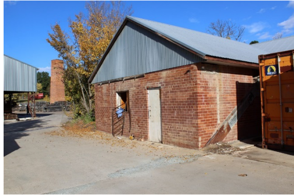
Figure 3.28 Substation/Control Room (Element 29). (Source: GML, 2017)
