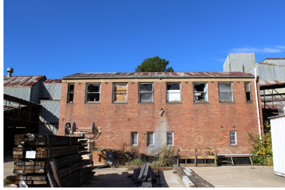
Figure 3.24 Amenities Block (Element 25). (Source: GML, 2017)
