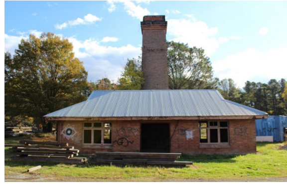
Figure 3.14 Fan House (Element 2) and Chimney Stack (Element 7) for Staffordshire Kiln. (Source: GML, 2017)
