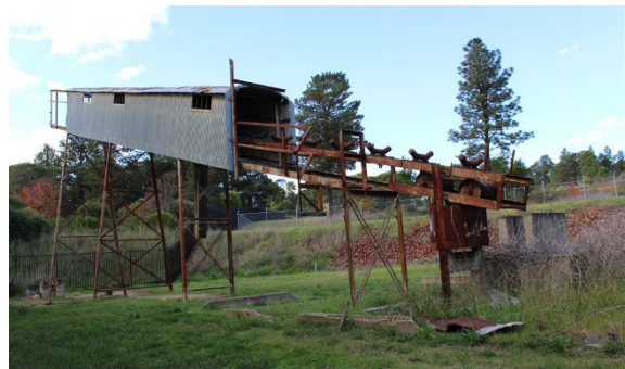
Figure 3.21 Elevator/Conveyor (Element 22). (Source: GML, 2017)
