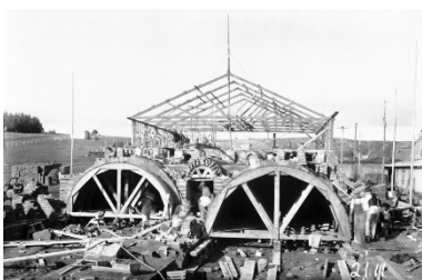
Figure 2.8 Hardy patent kiln 1 under construction, c1926. (Source: NAA, A3560, 2111)
