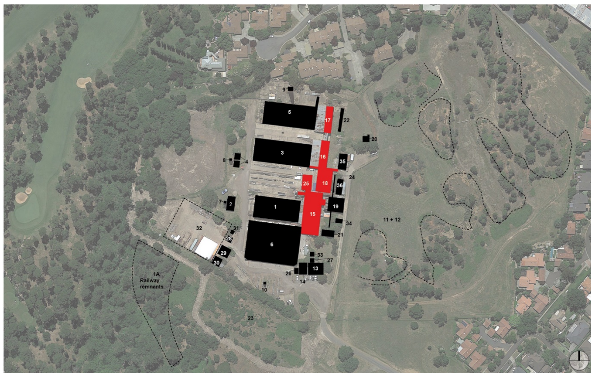
Figure 3.16 Location of the machine bays and workshop at the site, shown in red. (Source: Google Earth with GML overlay, 2017)
