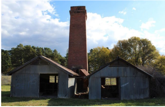
Figure 3.13 Fan Houses (Element 4) and Chimney Stack (Element 8) for Hardy Patent Kiln 1. (Source: GML, 2017)
