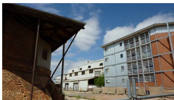
Figure 2.43 Former Hoffman works at Brunswick, 2010. (Source: Lovell Chen, 2010, Canberra Brickworks CMP, p 189)
