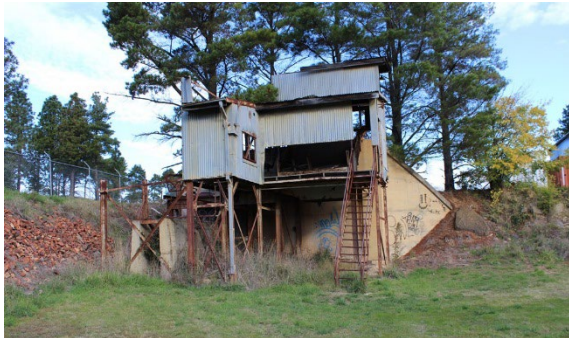
Figure 3.18 Primary Crusher House (Element 20). (Source: GML, 2017)
