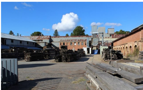
Figure 3.37 View east over the first brickyard toward the Amenities Block (Element 25). (Source: GML, 2017)
