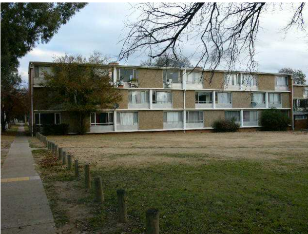
Image 5. Northbourne Flats. Typical two-bedroom blocks. (Source Milton Cameron 2011)
