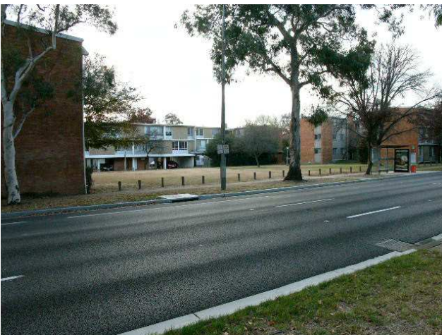
Image 2. Northbourne Flats. View from Northbourne Avenue looking north-west. (Source Milton Cameron 2011)
