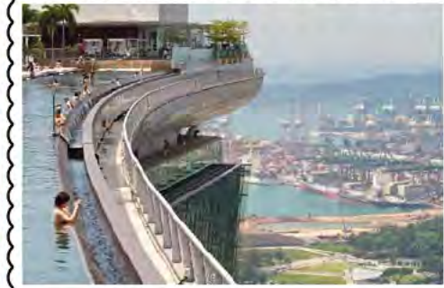
Infinity pool edge with maintenance pathway below
