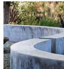
CURVED CONCRETE SEAT WALLS
