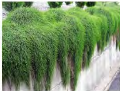
Precast concrete planter boxes
