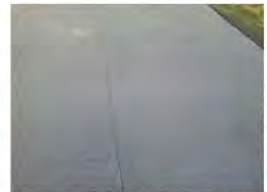
Concrete coloured sawcut - ground floor
