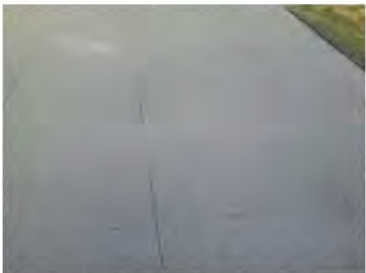
Courtyard paving - concrete coloured sawcut
