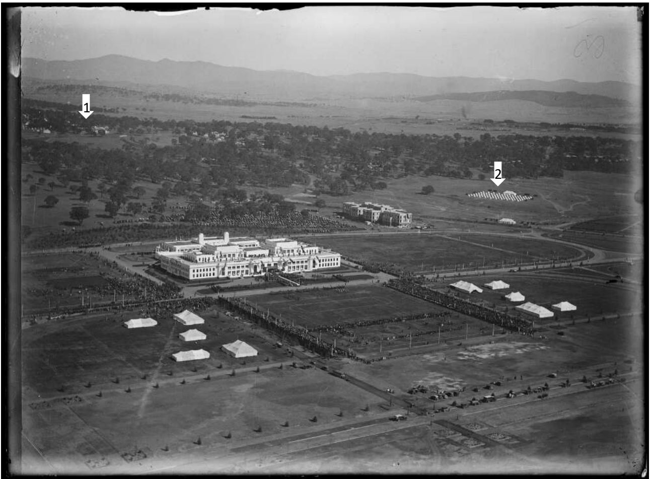
Figure 6: Aerial view of the opening of the Provisional Parliament House, 7 May 1927: (1) Capitol Hill with workers tents visible, (2) The temporary servicemen's camp (NLA n.d.).
