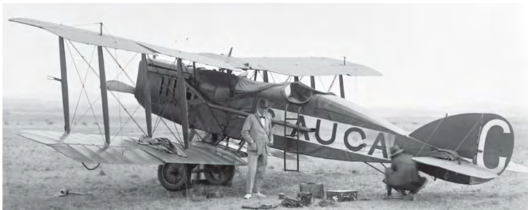
ABOVE: Colonel Percy Owen at the Aerodrome site inspection, 15 February 1923.
