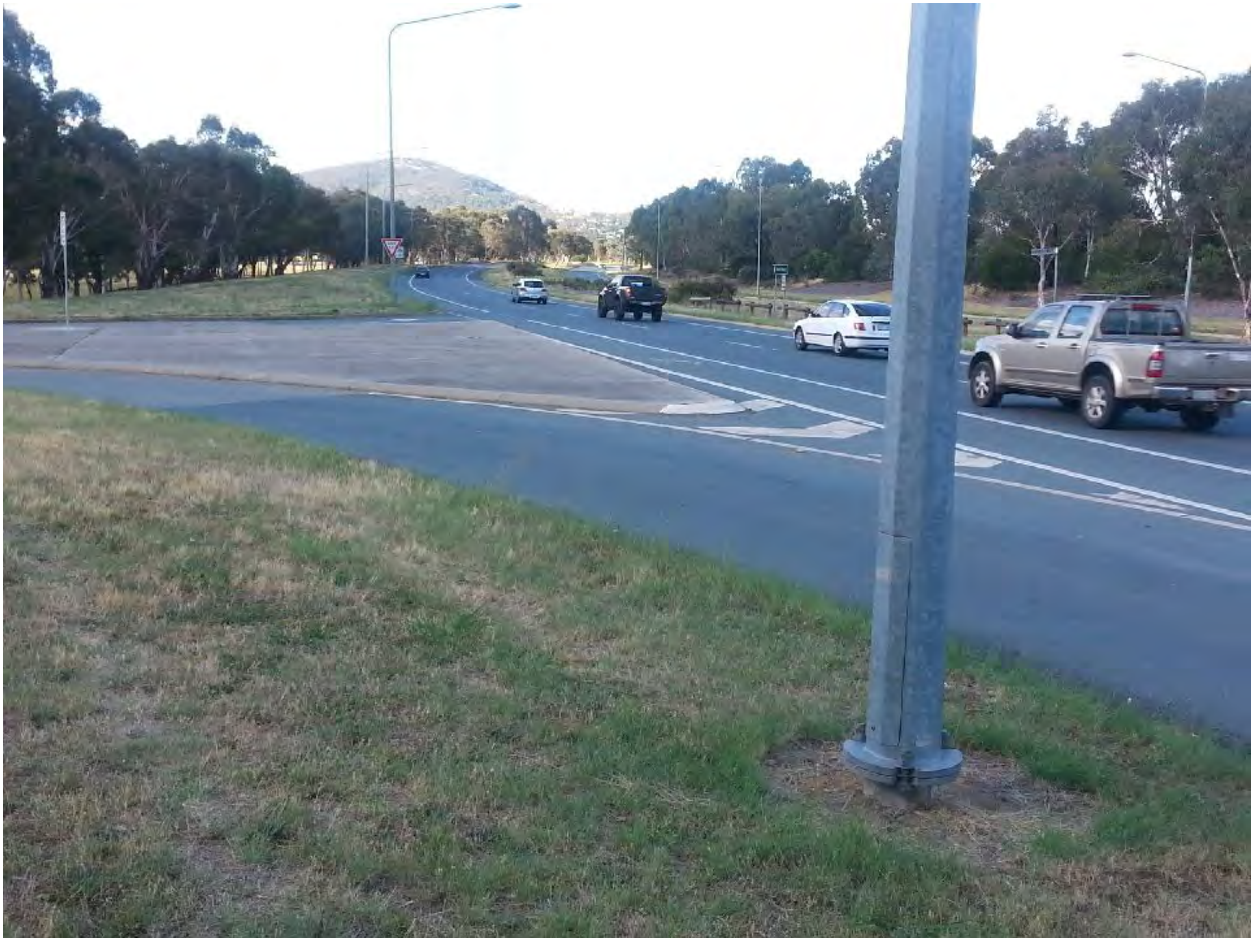
Figure 4: Drakeford Drive looking north from south of Mortimer Lewis Drive
