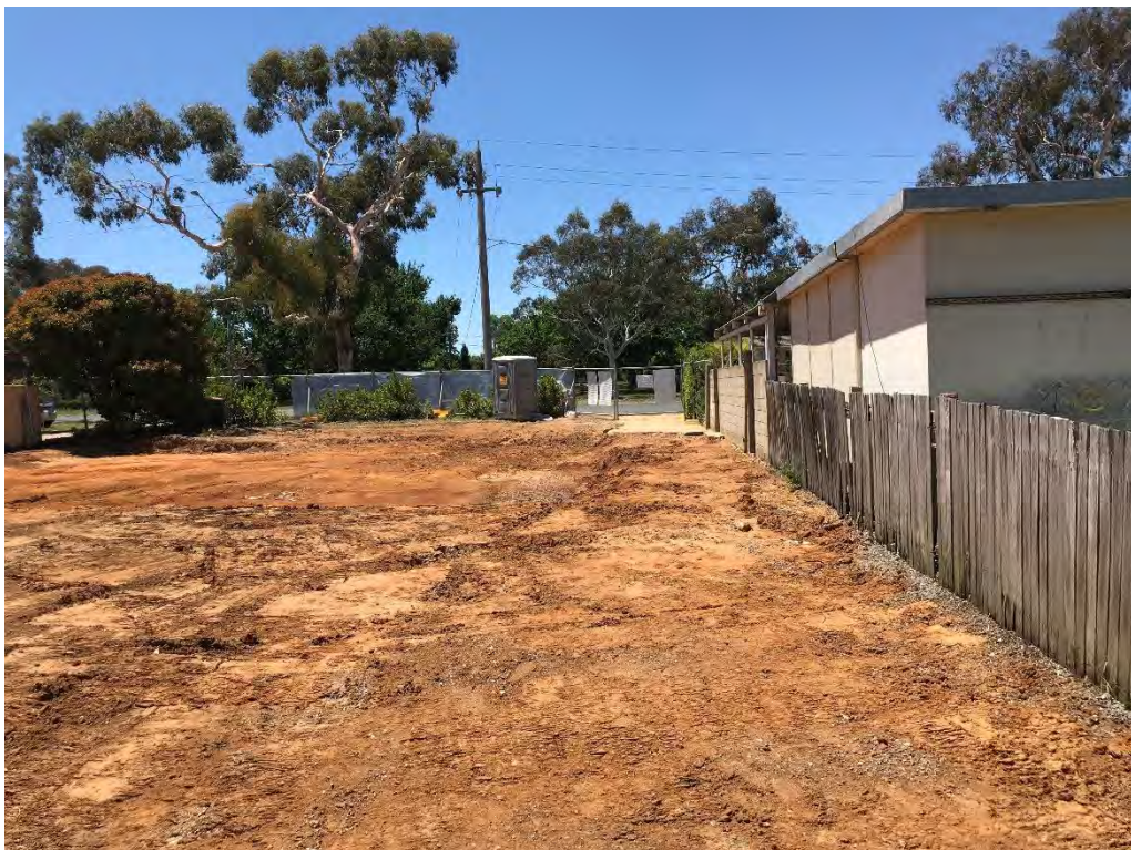
Figure 2 Site overview of demolition footprint.
