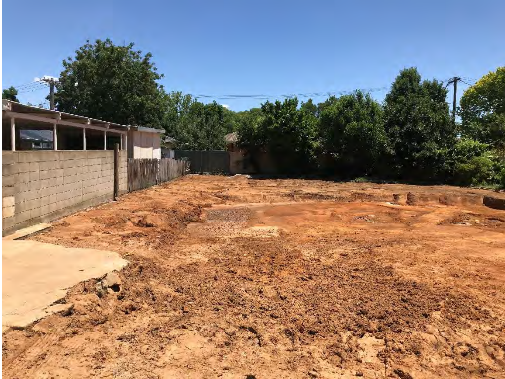
Figure 1 Site overview of demolition footprint.
