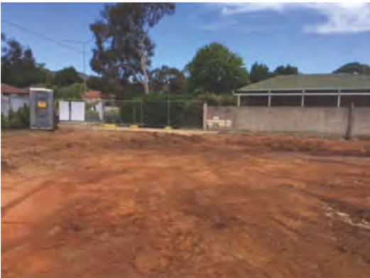
Cleared area of the demolition zone
