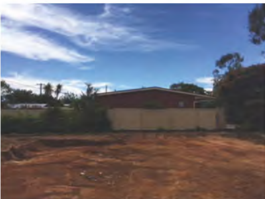
Cleared area of the demolition zone
