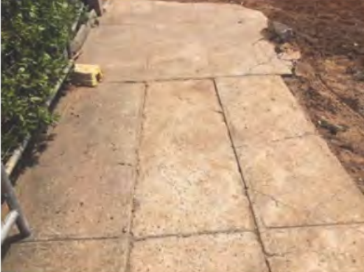
Driveway outside the demolition zone
