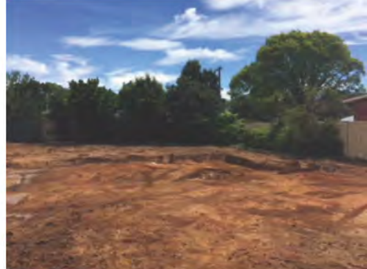
Cleared area of the demolition zone
