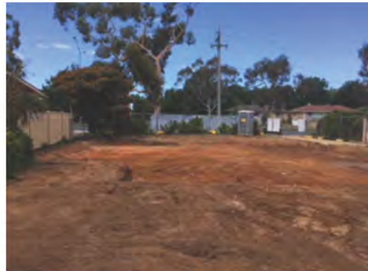
Cleared area of the demolition zone
