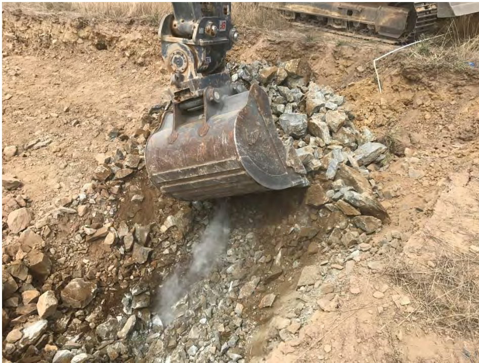
Figure 2: Test pit excavation within the western corner of the [redacted]
