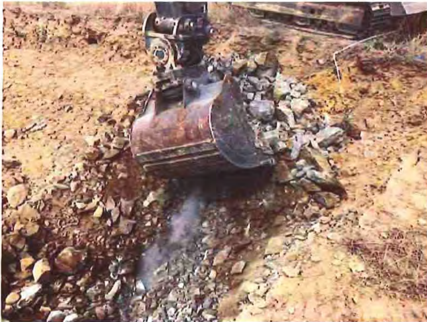
Figure 2: Test pit excavation within the western corner of the Block [REDACTED]
