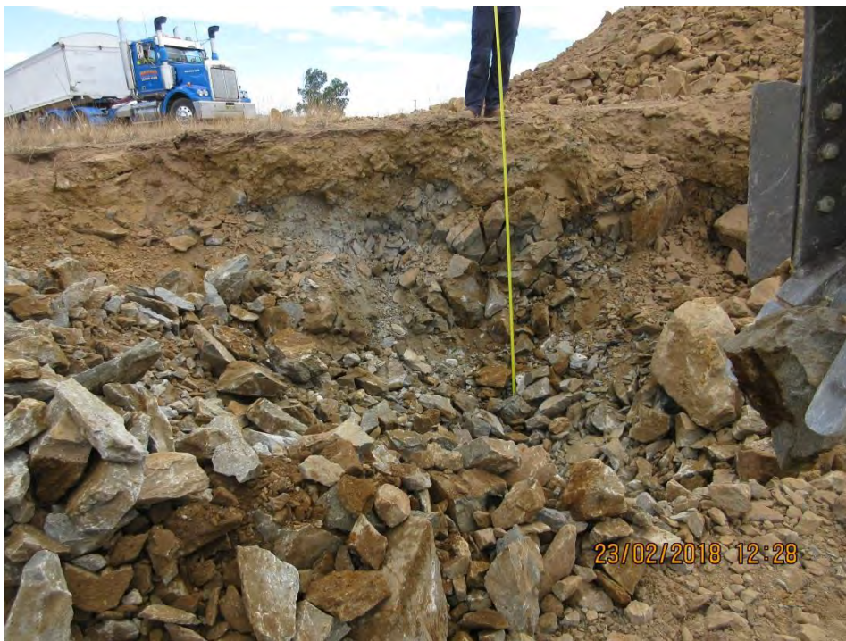
Figure 3: View of the side boundary and test pit excavation profile
