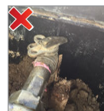
No clearance for Ball valve
