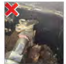
No clearance for Ball valve
