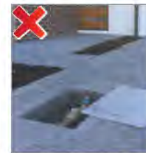
In driveway (unapproved)
