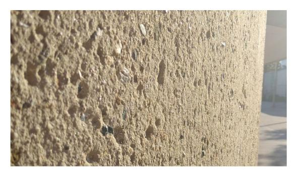
Figure 11 Detail of exposed aggregate sandblasted finish to concrete walls, (ACT Heritage, 2021)
