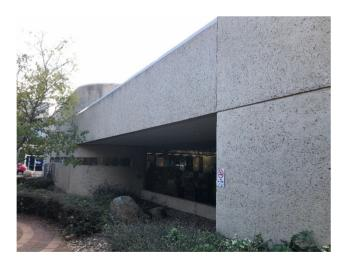
Figure 13 Recess along the southern facade for protected full height glazing, (ACT Heritage, 2020)
