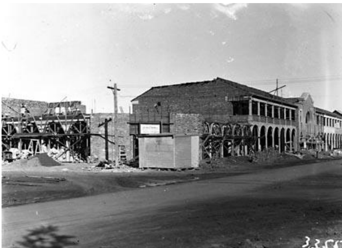
Figure 27. Sydney Building? under construction, 1927
