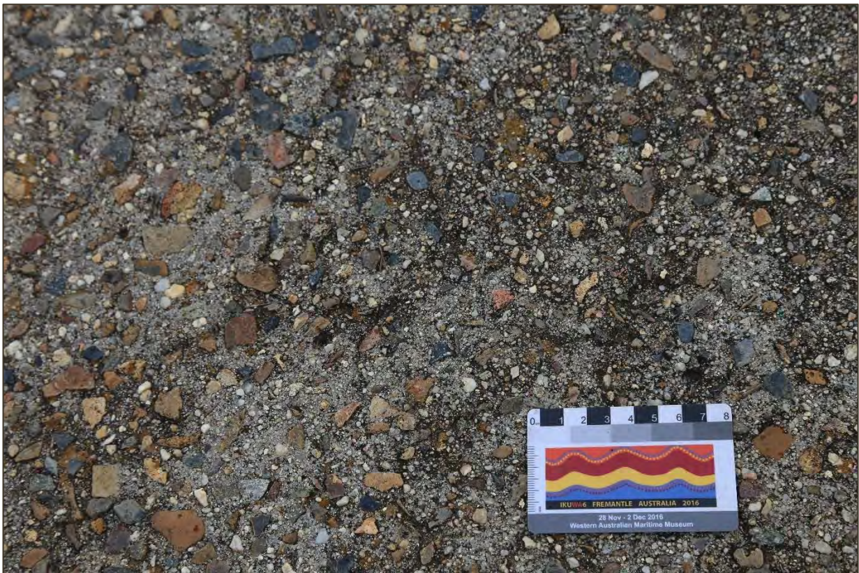
Figure 37. A fragment of the concrete curb associated with the previous car park and driveway of the previous Downer Club and CSDO (top) located at the northwest corner of the study area, and a close-up image of its poorly-sorted gravel and sand aggregate on its surface (bottom).
