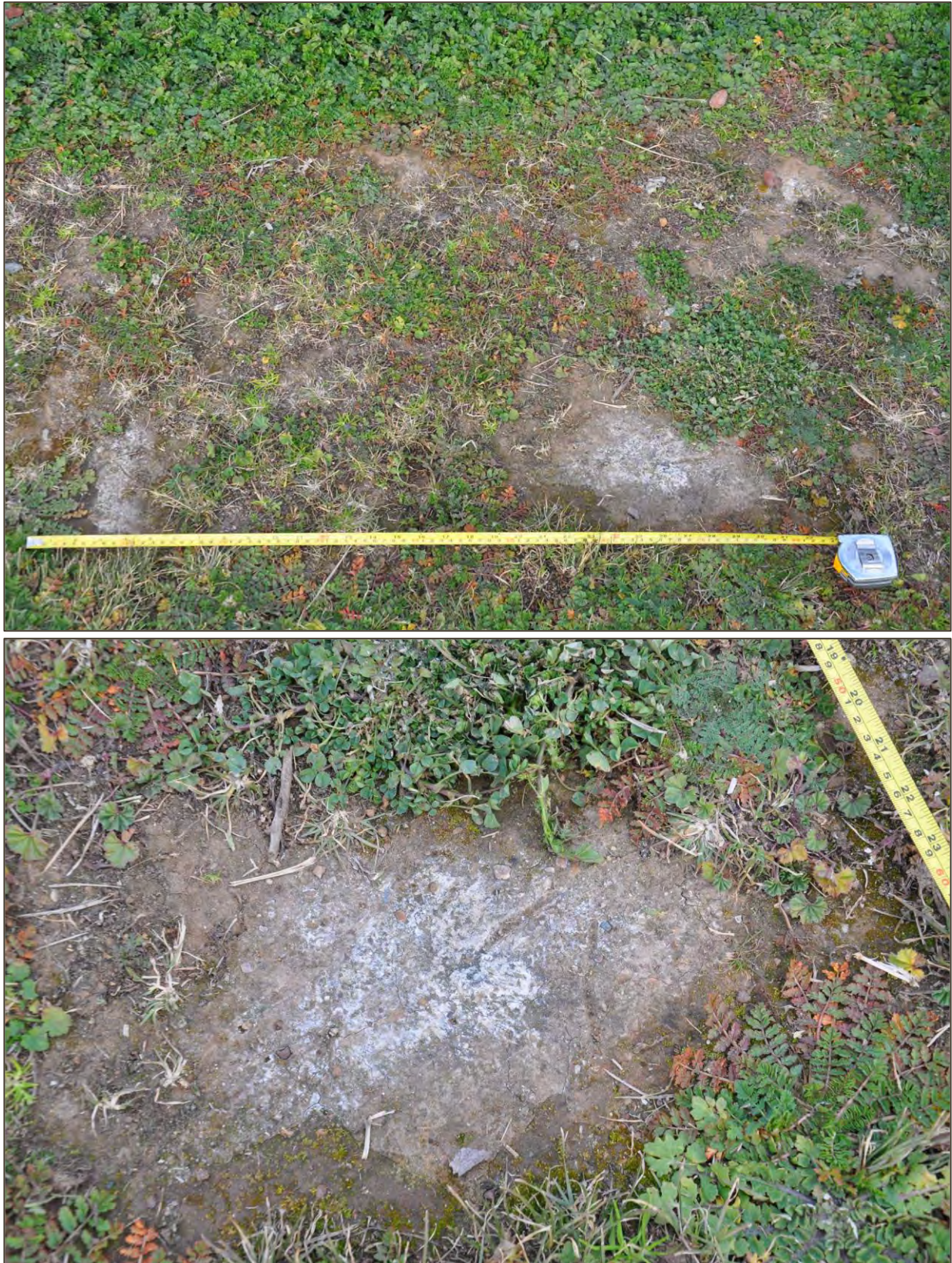
Figure 39. One of the four concrete, whitewashed, lockspits (top) marking the southeast corner of the landing ground of the former Canberra Aerodrome presently located within the grounds of the Dickson Wetland (c.400 m southeast of the study area), and a close-up view of its exterior surface (Source: Kent and Oglethorpe 2020, Attachment 2).
