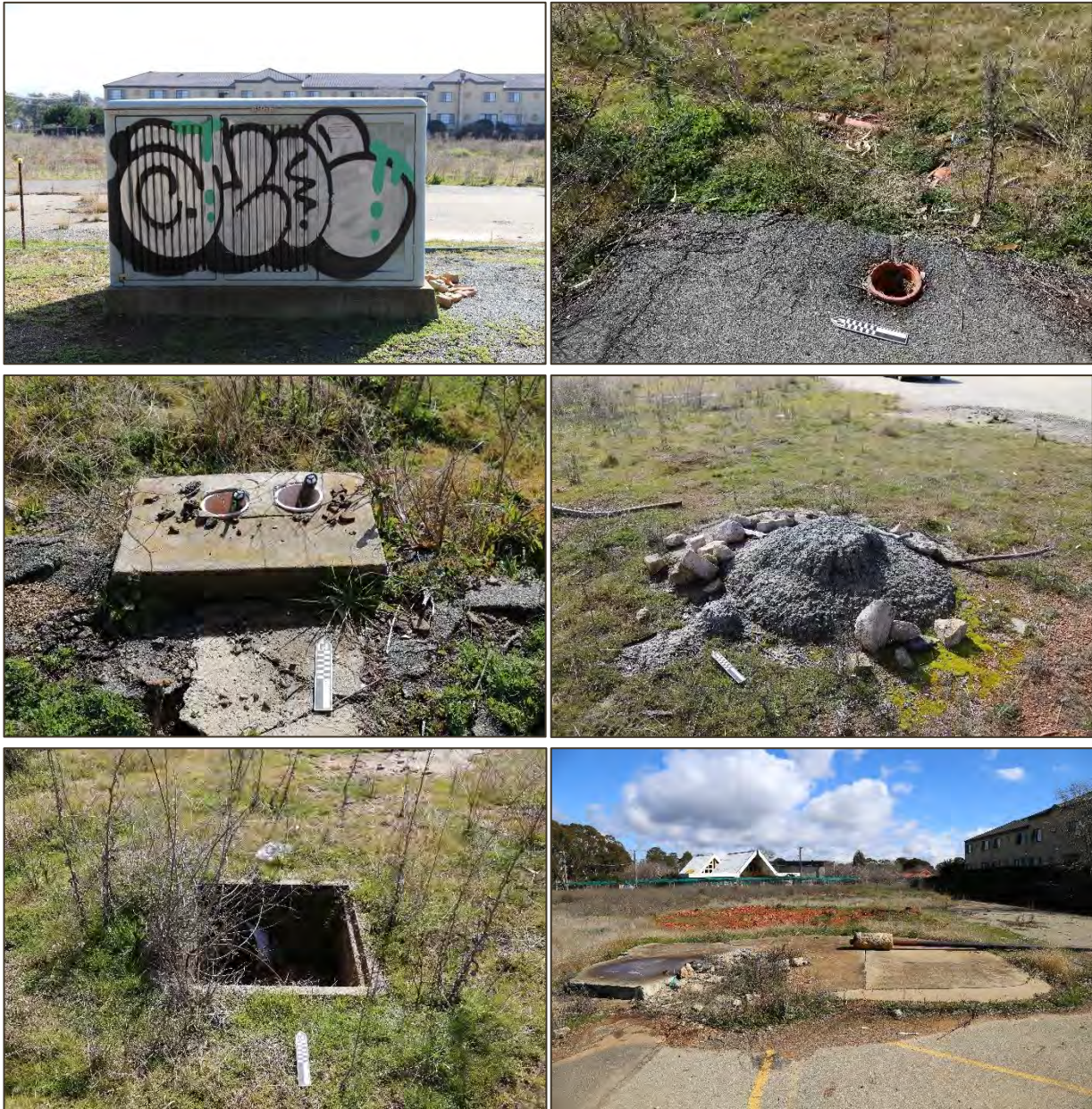
Figure 33. Various building and infrastructure remains associated with the Downer Club and CSDO variably distributed across the entire surface of the study area. These structures and remains include the substation electrical box and concrete pedestal installed in 1993 (top, left), a sub-surface ceramic stormwater pipe (top, right), a sub-surface electrical wiring and easement (middle, left), concrete and brick structural remains (middle, right), sub-surface stormwater drainage and access (bottom, left) as well as concrete curb and pedestrian pavement remains (bottom, right).
