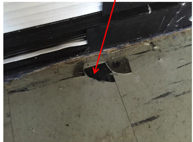
Photograph 6: Ground level, asbestos containing vinyl floor tiles and blackjack adhesive (exposed) beneath carpet throughout.
