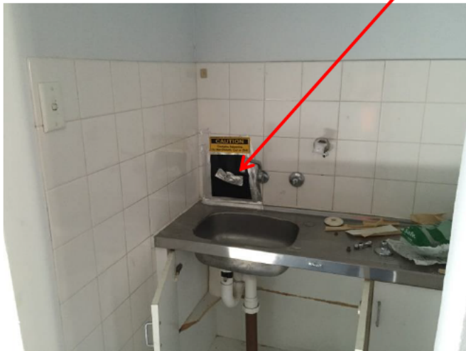
Photograph 11: Level 1, kitchenette, asbestos lagging (covered and labelled) to hot water pipes.
