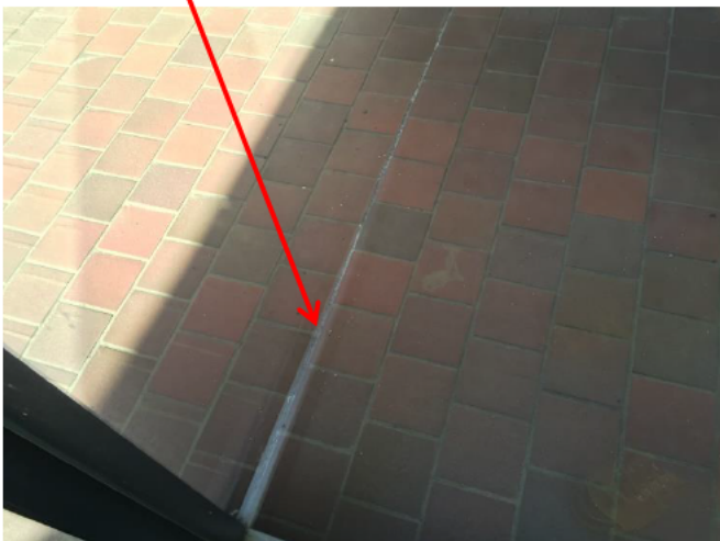
Photograph 15: Level 2, exterior balcony, asbestos containing putty used as sealant to expansion joints.
