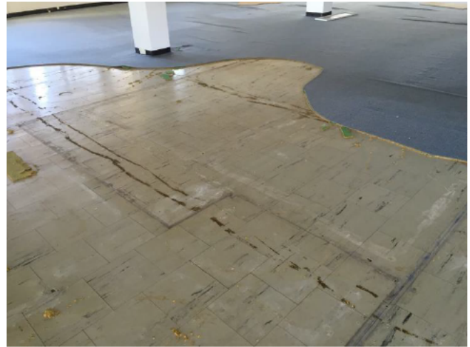
Photograph 10: Level 1, exterior balcony, asbestos containing sealant to expansion joints / tile cracks.
