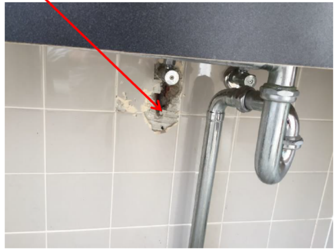
Photograph 12: Level 1, male bathroom, asbestos lagging to hot water pipes chased into wall masonry.
