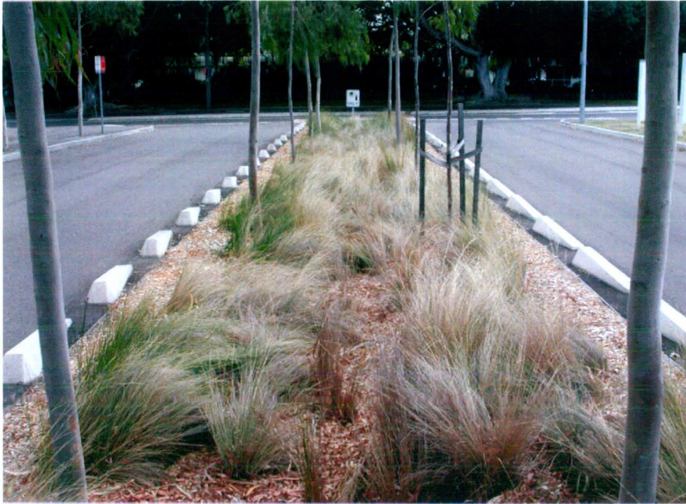
Figure 18 Street scale linear bioretention system – Victoria Park, Sydney
