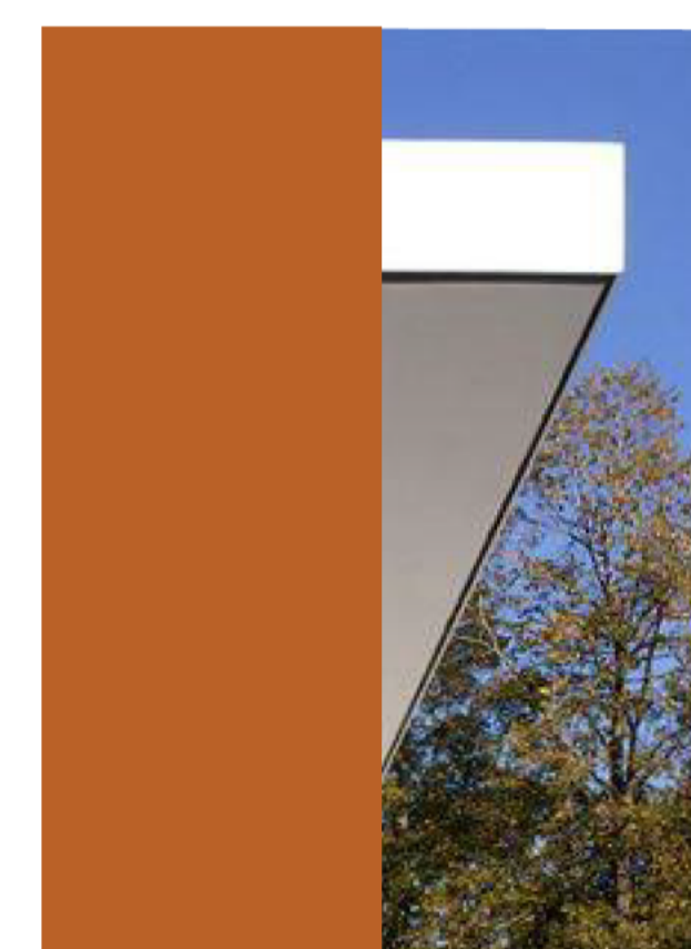
CLD 2 ALUMINIUM CLAD FAIRVIEW VITRADUAL DESERT ORANGE AWN 1 ALUMINIUM CLAD AWNING WITH WHITE FC SOFFIT FAIRVIEW VITRADUAL SNOW WHITE
