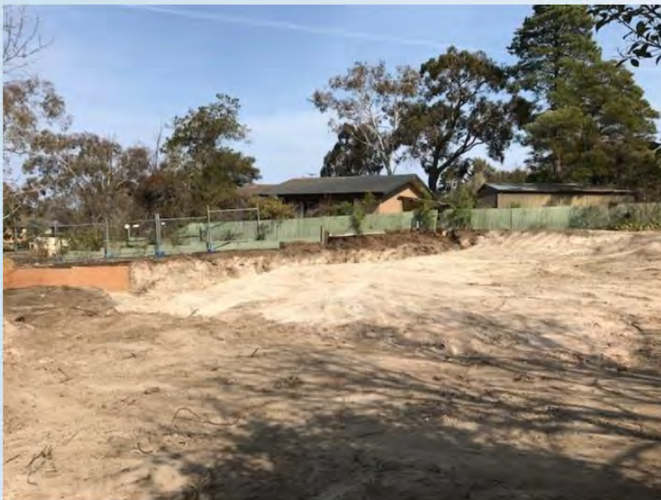
Photograph 2 – Dwelling footprint ground surfaces, taken from Northern side of the site.
