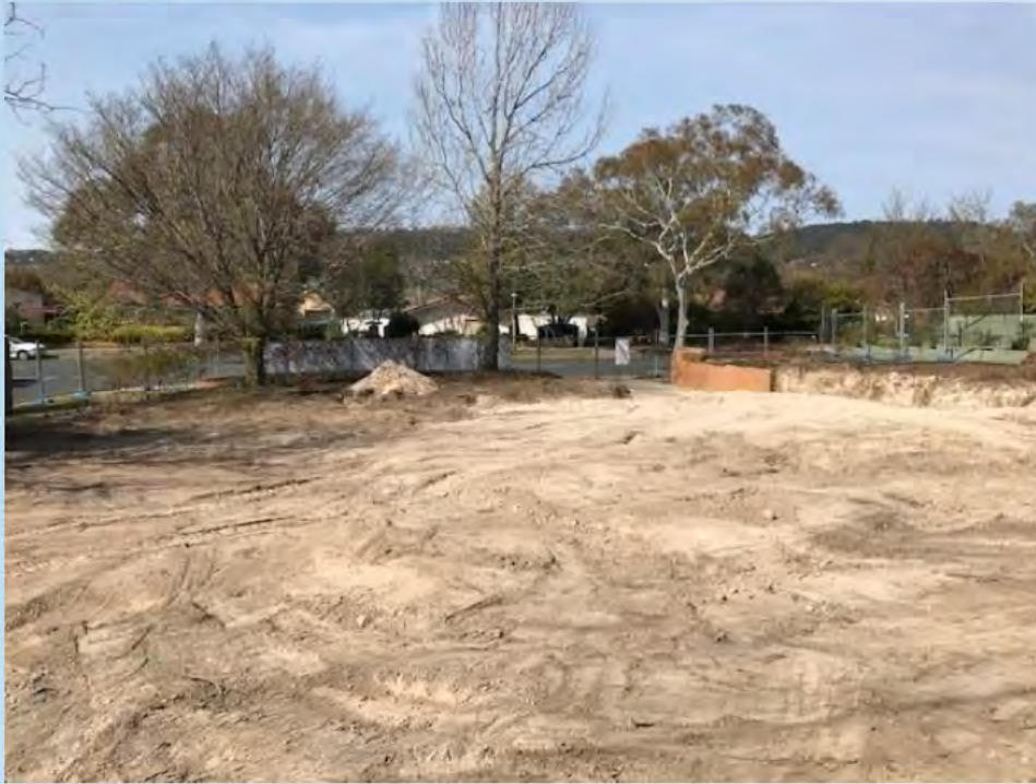
Photograph 1 – Dwelling footprint ground surfaces, taken from Western side of the site.
