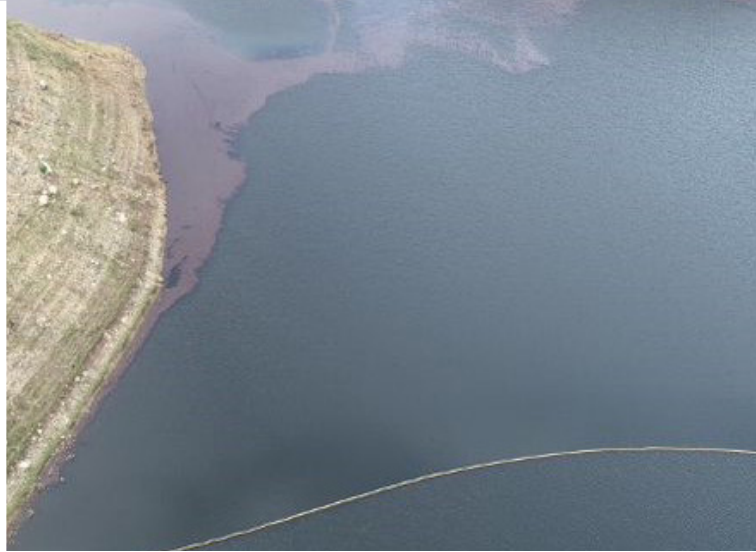
One of three silt curtains installed in Corin Dam reservoir during the Orroral Valley Fire — February 2020
