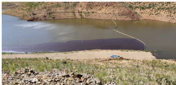
A silt curtain slowed and trapped sediment and small debris in the Corin Dam reservoir following the Orroral Valley Fire. Large debris that was trapped by the curtain was manually removed from the reservoir — April 2020.
