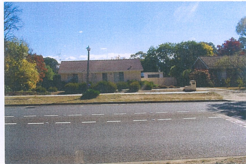
ADJOINING ORIGINAL HOUSE TO THE NORTH (55 AINSWORTH STREET) PAINTED MASONRY WALLS TO BE RECALLED WITHIN PROPOSED DEVELOPMENT.
