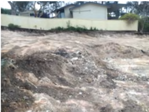
Cleared area of the demolition zone
