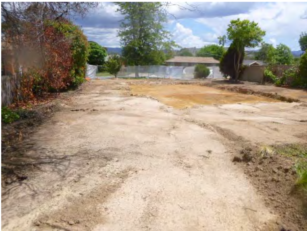
Figure 2 Site overview of demolition footprint.
