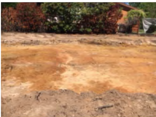
Cleared area of the demolition zone
