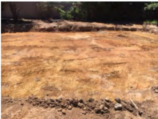
Cleared area of the demolition zone
