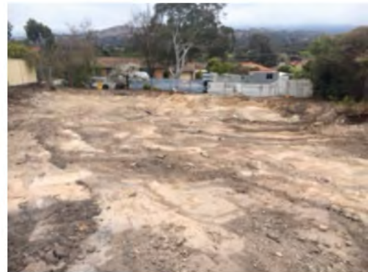
Cleared area of the demolition zone
