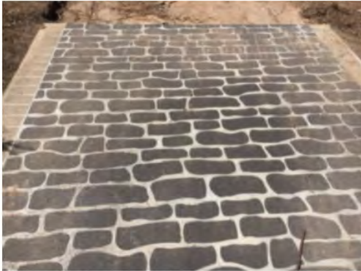
Driveway outside the demolition zone
