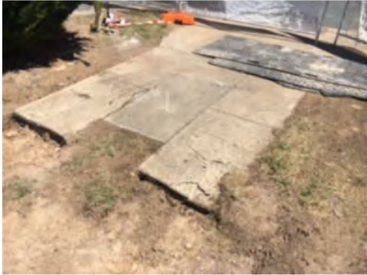
Driveway outside the demolition zone
