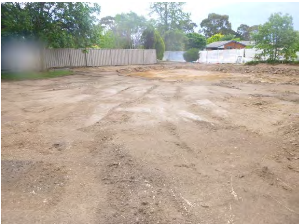
Figure 2 Site overview of demolition footprint.
