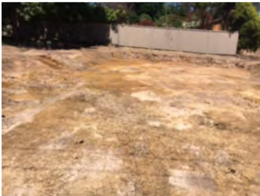
Cleared area of the demolition zone
