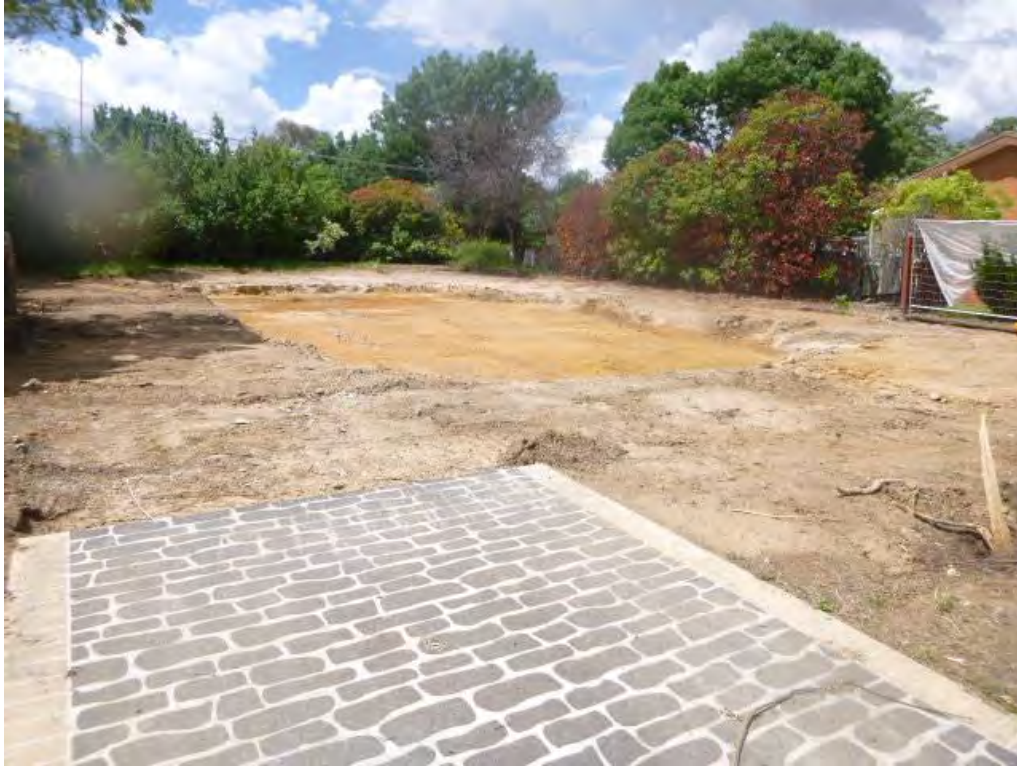
Figure 1 Site overview of demolition footprint.
