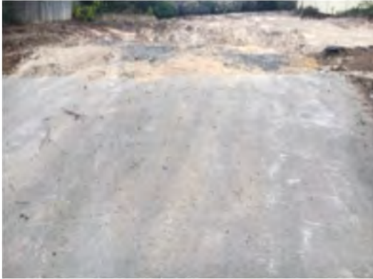
Driveway outside the demolition zone
