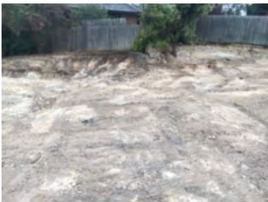
Cleared area of the demolition zone
