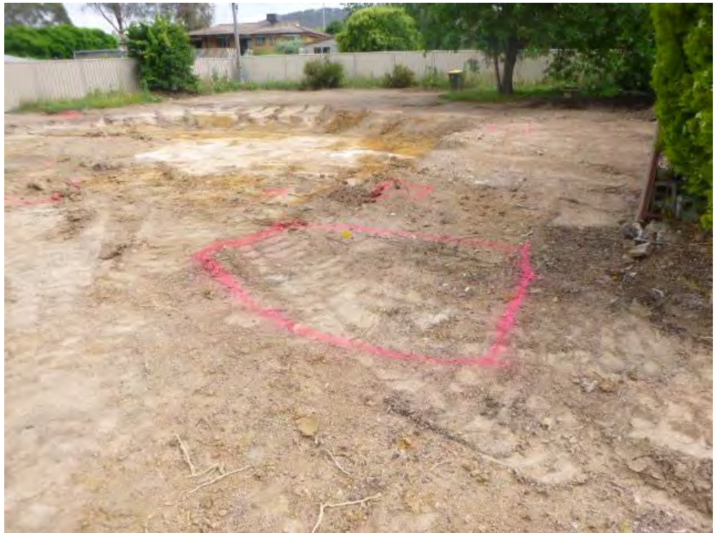
Figure 8 View from the south-eastern corner of the demolition area to the northern boundary. Photograph taken after soil scrape - painted areas are visual fibre cement sheet.
