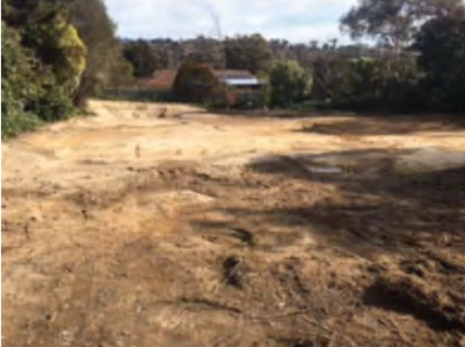
Cleared area of the demolition zone
