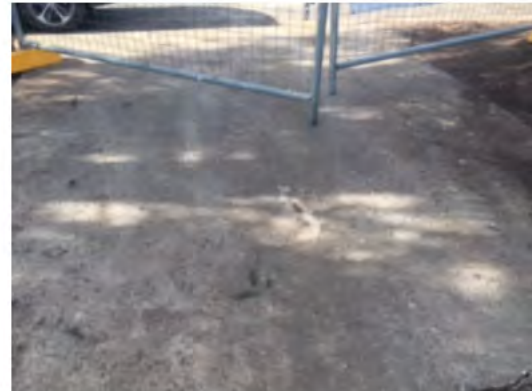
Driveway outside the demolition zone
