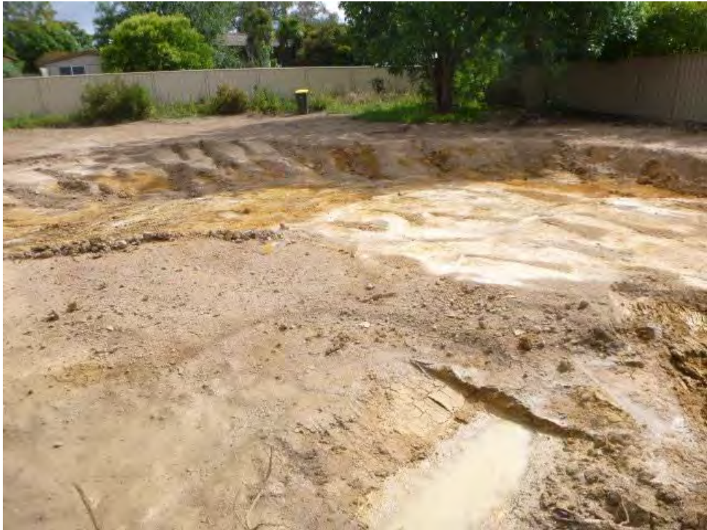
Figure 9 Overview of the first Hot Spot scrape.
