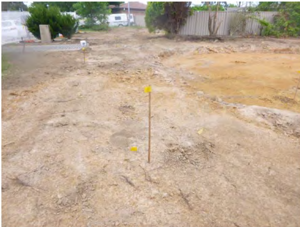
Figure 7 Soil validation sample location/s (from the left) view from the southern corner of the housing footprint to the western boundary: S01, S02, S12, S03, S04 and S11. Note remaining colour bond fence separating 45 and 46 McDermott Street, Kambah.
