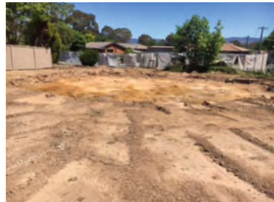
Cleared area of the demolition zone
