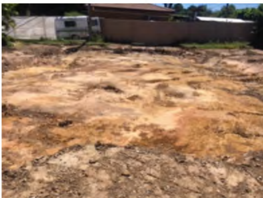
Cleared area of the demolition zone
