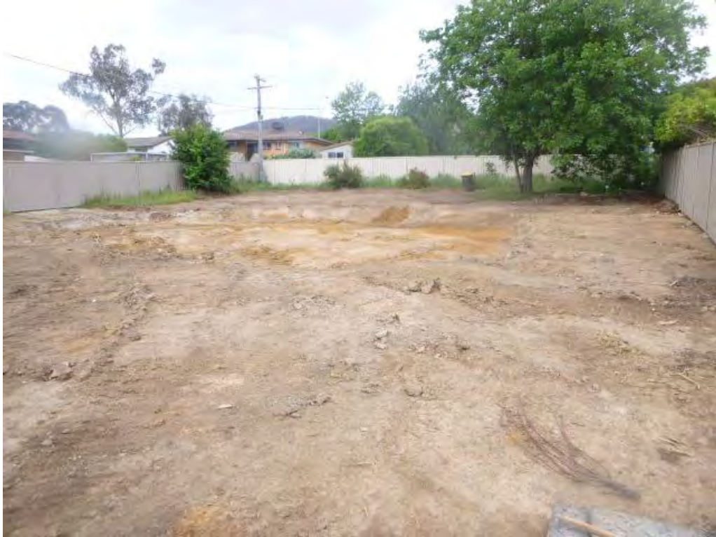
Figure 1 Site overview of demolition footprint.
