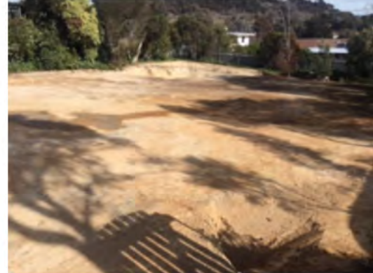
Cleared area of the demolition zone
