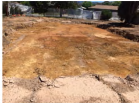
Cleared area of the demolition zone
