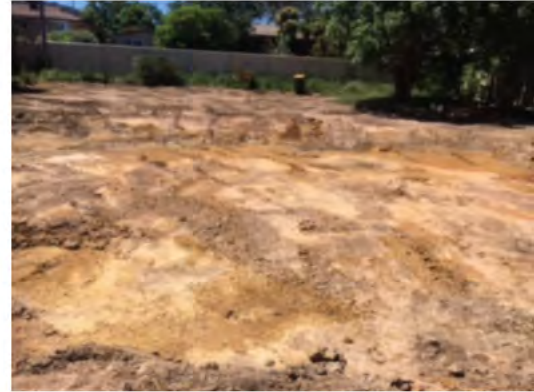
Cleared area of the demolition zone
