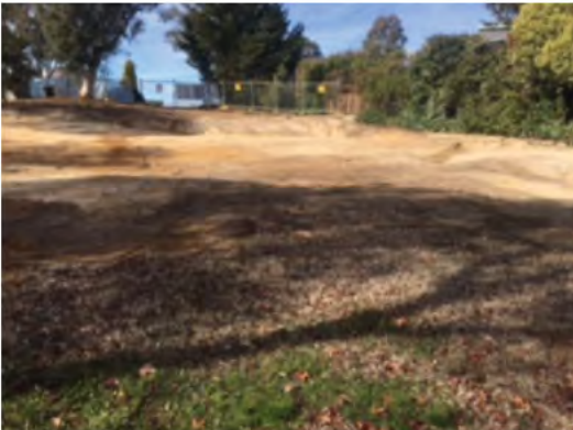
Cleared area of the demolition zone
