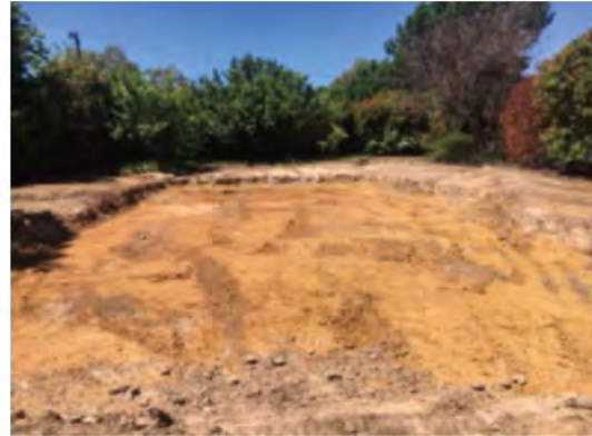
Cleared area of the demolition zone
