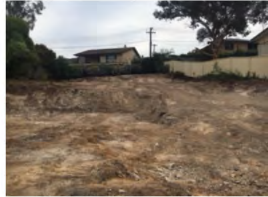
Cleared area of the demolition zone
