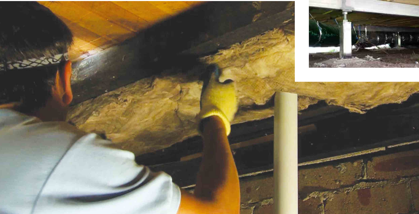
Installing underfloor insulation
