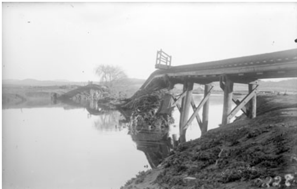
Figure 6 Railway bridge over Molonglo River showing flood damage after July 1922 floods (NLA: A3560, 228)
