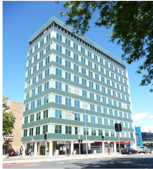
Image 5 former MLC Building north and west facades (ACT Heritage, 2014)
