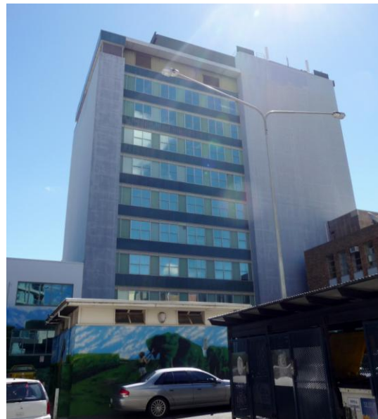
Image 6 former MLC Building east and south facades (ACT Heritage, 2014)
