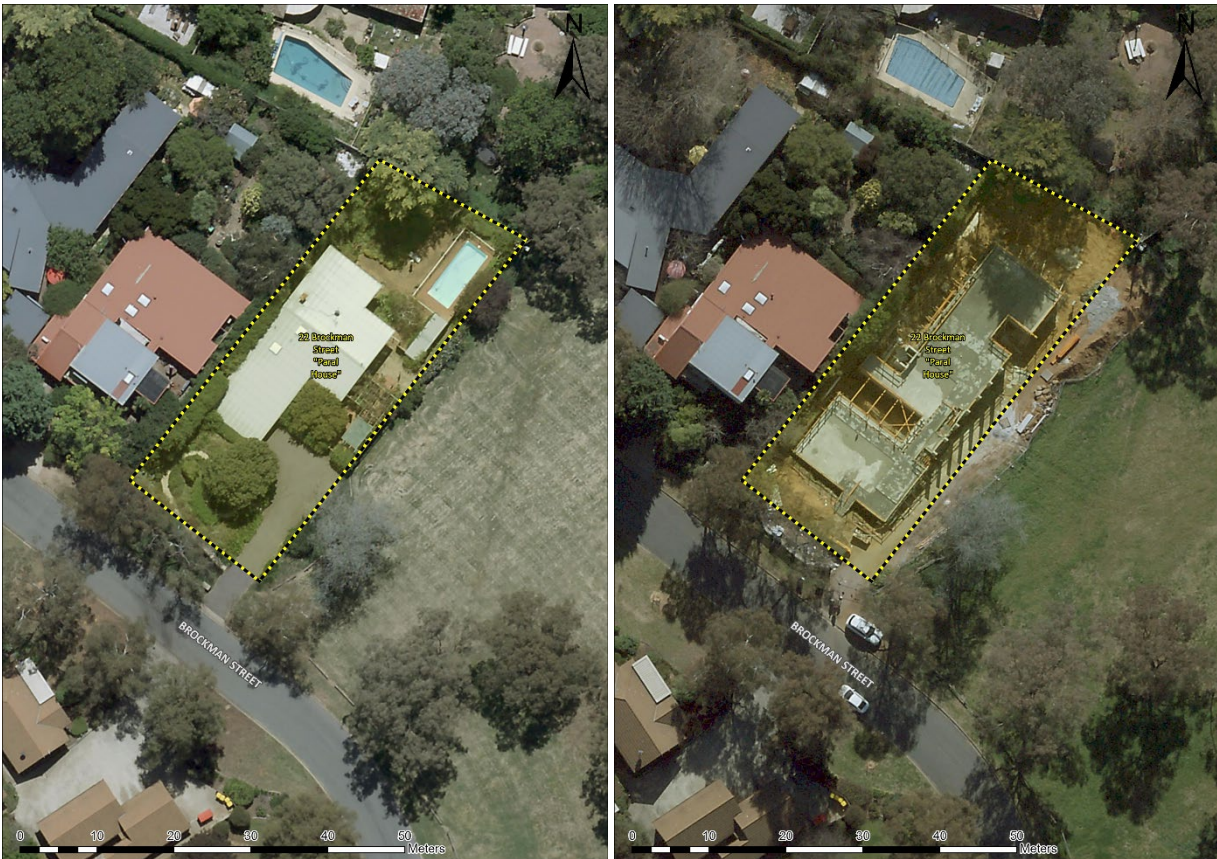
Image 1 Paral House site boundary – left in 2021 with the original house, right in 2022 with the new house mid-construction.
