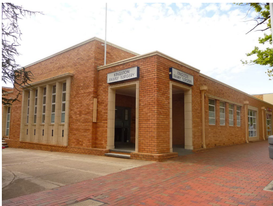
Figure 2 Former Kingston Post Office building as seen from the corner of Giles and Jardine Street. Minor modifications to the building are observable, including the replacement of the stylised lettering (ACT Heritage Unit, October 2021).
